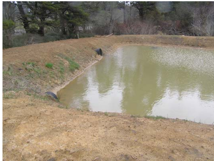
Tailwater Recovery System
