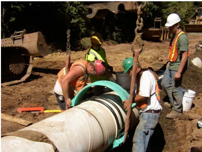
Figure 3. EFID CLPP “Lower Phase” work during 2007 ( new system ).
