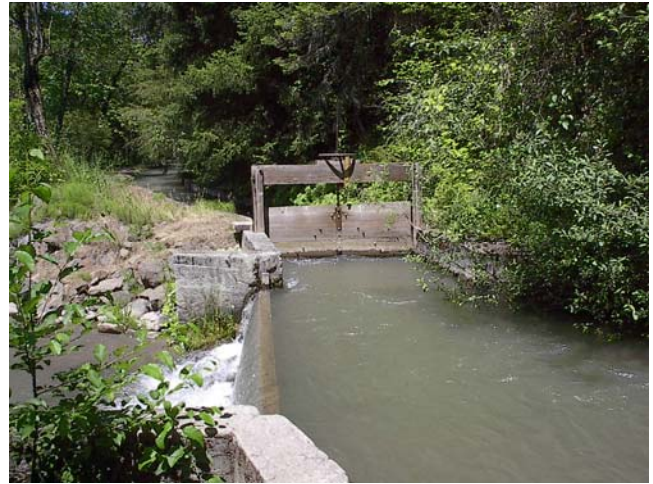
Figure 4. Eastside Lateral Diversion and old fish ladder (to be removed in 2009 to complete project).
