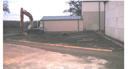
Above - Local Linn/Benton detention recreation yard excavation at sunset.
