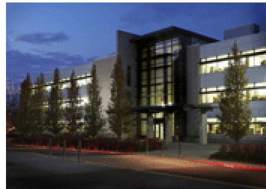
North Mall Office Building
