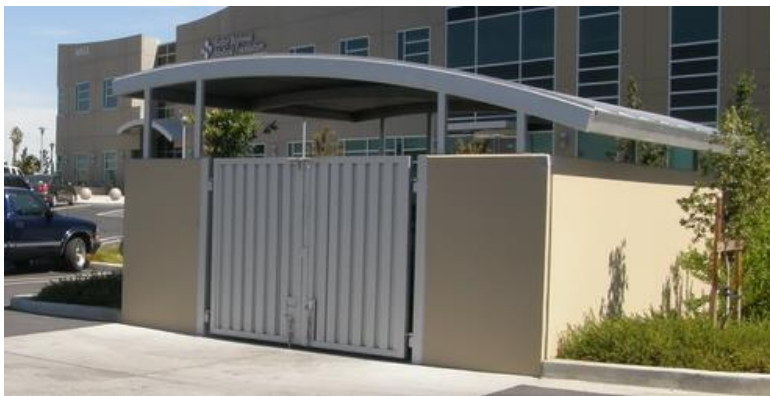
Figure 4: Sloped roof for storm water diversion and adjacent landscaping
