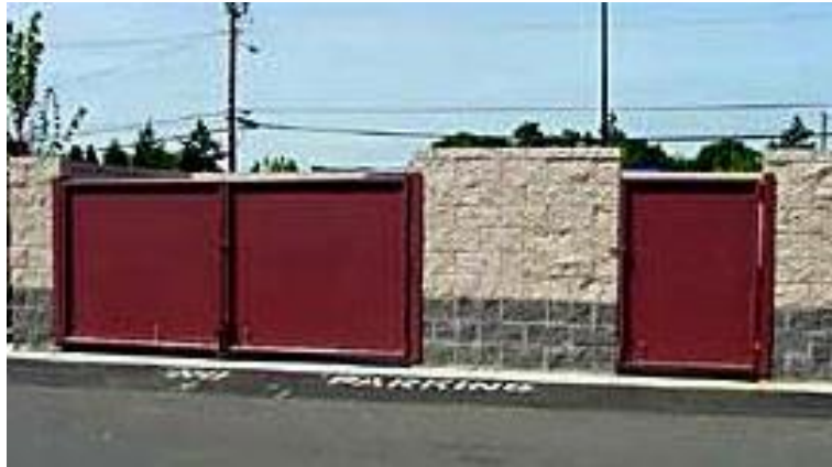
Figure 5: Separate pedestrian entrance
