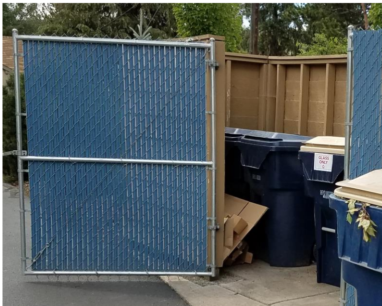
Figure 3: Receptacle with walkway less than 32 in. and access blocked by uncontained cardboard
