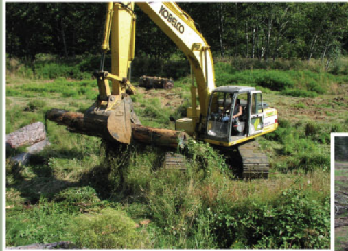
Figure 8. Placing large wood in the Anderson Creek channel and floodplain.
