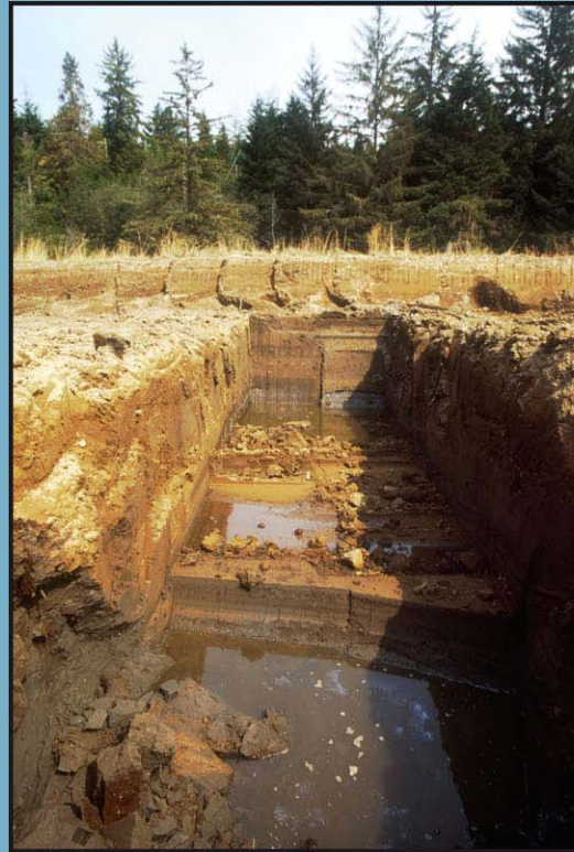
Figure 6. Trench used on-site for rapid dike-material disposal.
