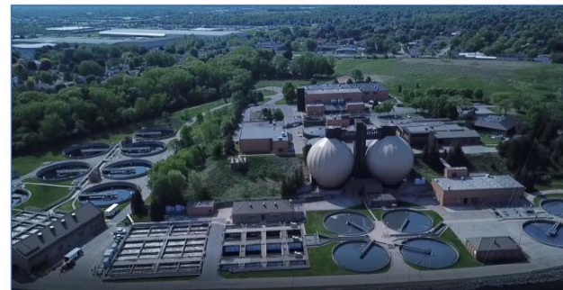
Photo 9: Biogas system, Appleton Wastewater Treatment Plant, Appleton, WI
