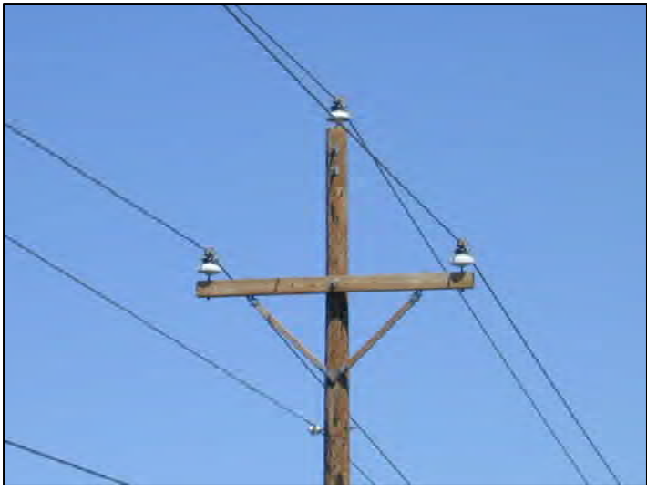
Three phase tangent, lowered 8-foot arm (Raptor-safe construction)
