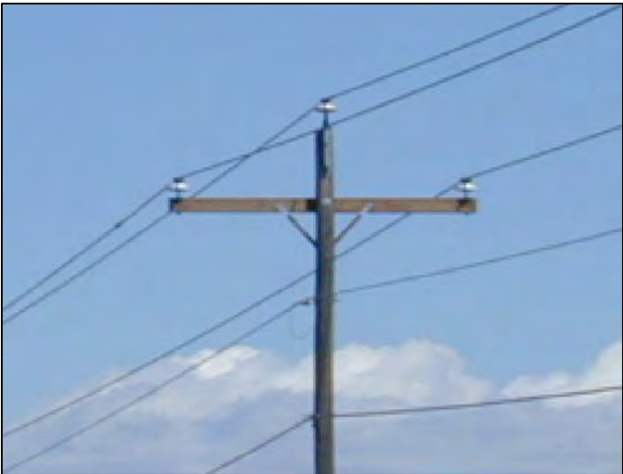
Three phase tangent, 10-foot arm (Raptor-safe construction)
