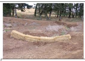
Straw bales are keyed into the soil in this low area to slow runoff water. The area will also be seeded heavily with grass seed, creating a grassed waterway.
