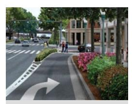
Right turn lanes allow motorists to move out of the through travel lanes and slow before turning from right the highway.
