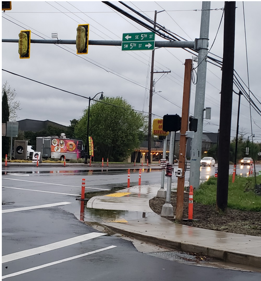
Figure 800-37: Water Accumulation at Curb Ramp
