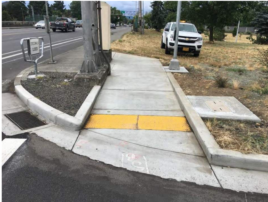
Figure 800-44: Curb Ramp System with a Directional Curb
