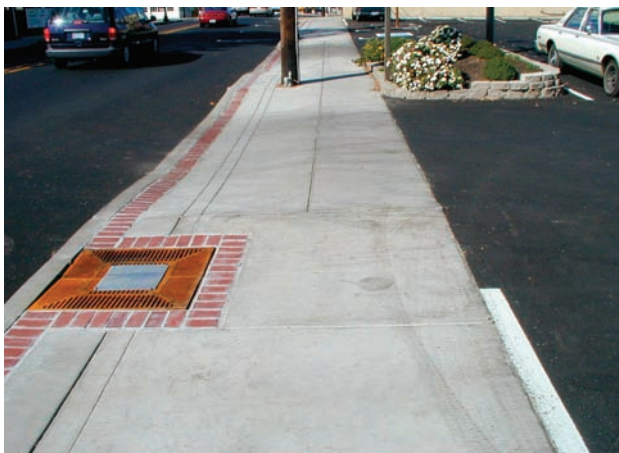
Dustpan style driveway approach improves pedestrian safety
