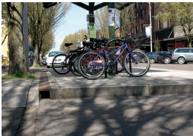
Slotted drain at retrofit curb extension
