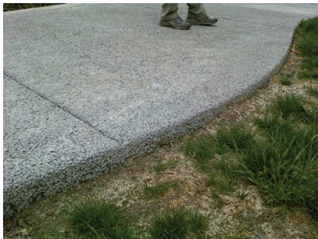
Concrete mix design is critical in pervious sidewalk to avoid a rough surface
