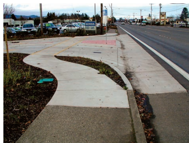
Commercial driveway with wrapped, level sidewalk and pork chop island
