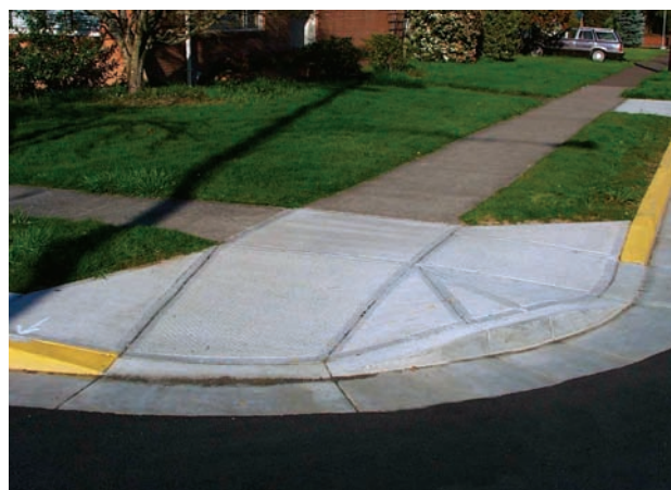
Ramp placement on separated sidewalk, NOTE: outside flares are not required.
