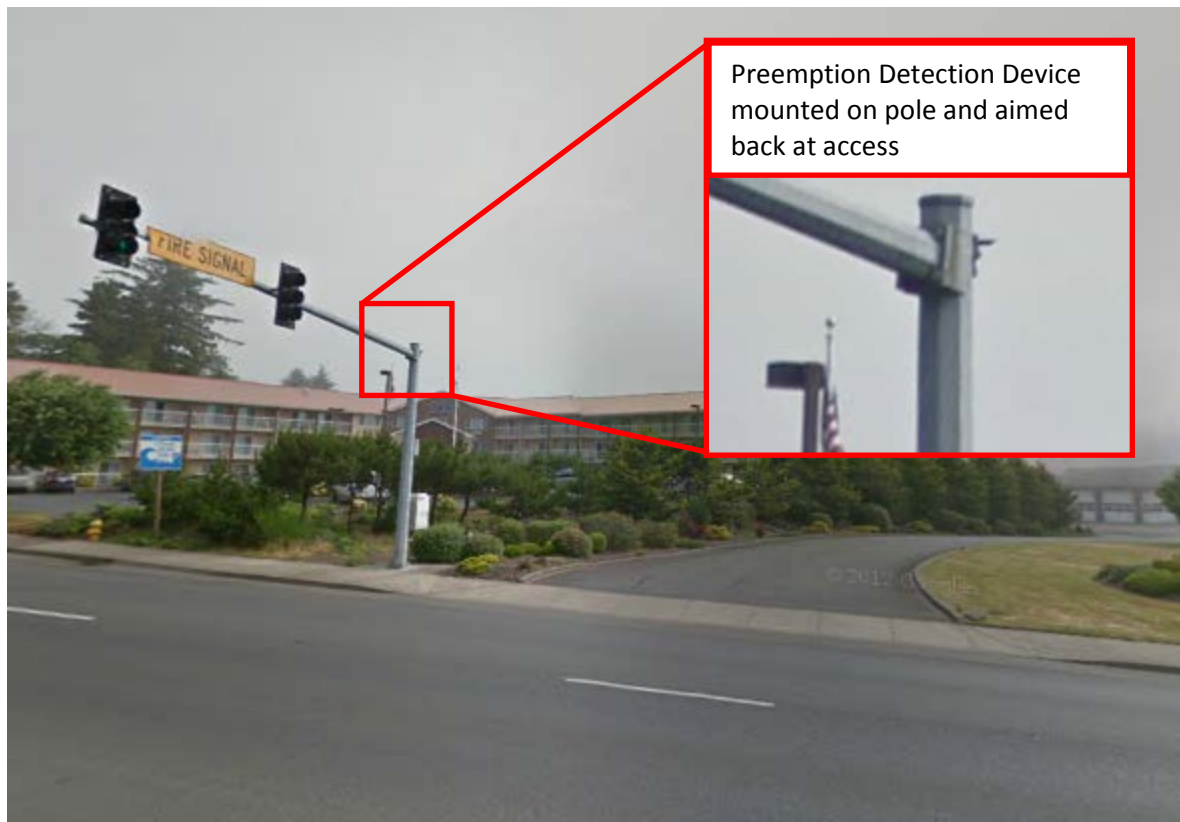
Figure 17-10 | Preemption Detection Device – Placement Example
