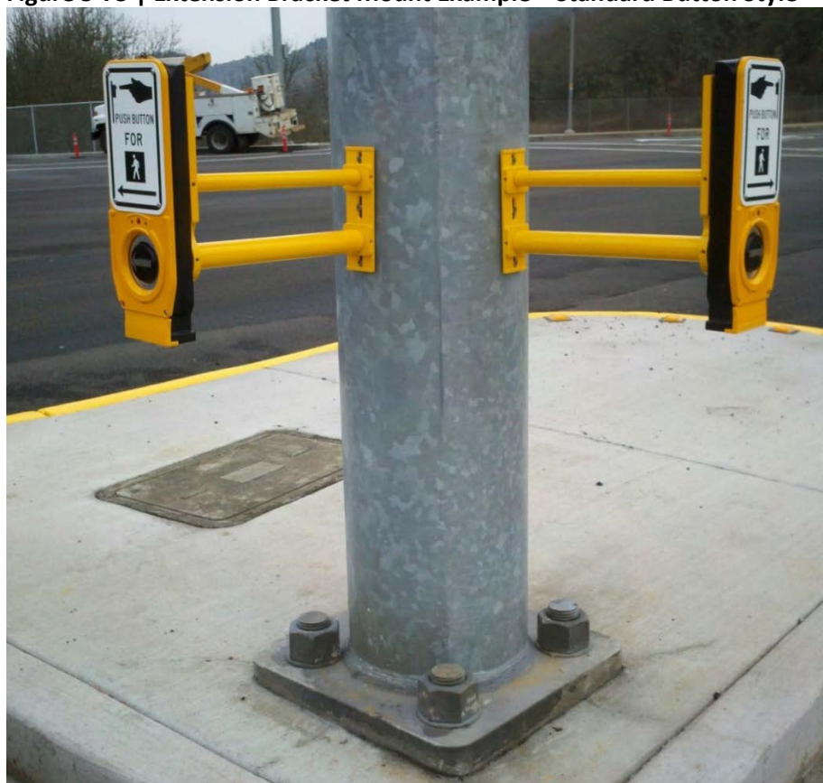
Figure 5-75 | Extension Bracket Mount Example – Standard Button Style
