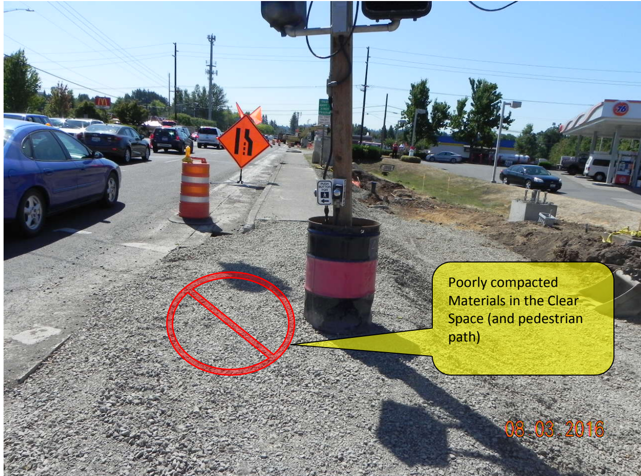
Figure 5-55 | Poorly Compacted Material Example
