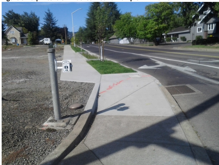
Figure 5-76 | Extension Bracket Mount Example – H-Frame
