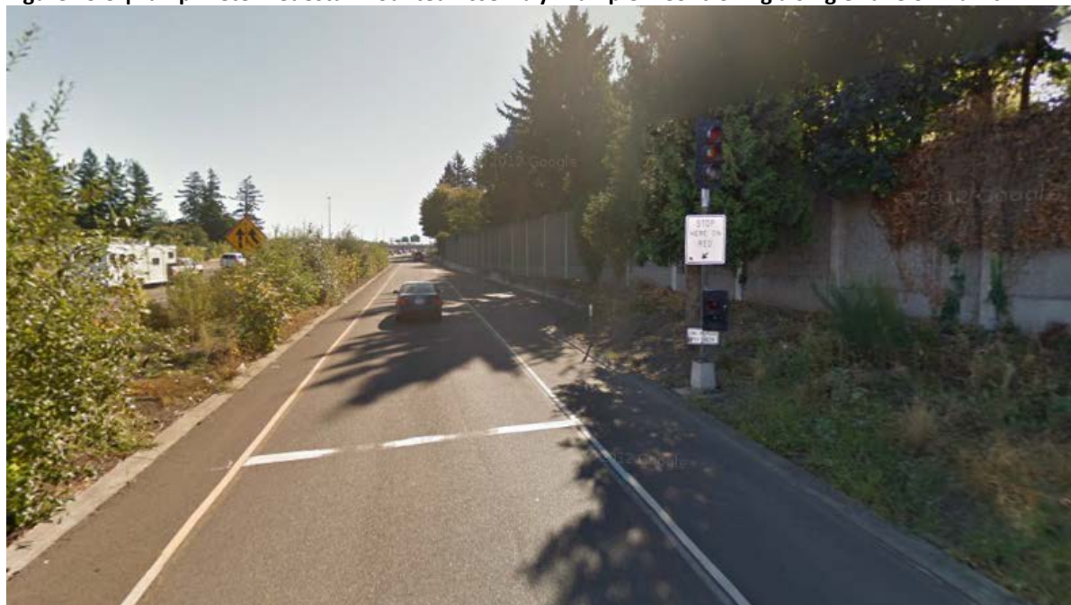
Figure 13-5 | Ramp Meter Pedestal Mounted Assembly Example – Controlling a Single Lane of Traffic
