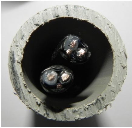
1" conduit w/2 loop feeder cables Does NOT exceed NEC max fill Does NOT exceed ODOT max fill
