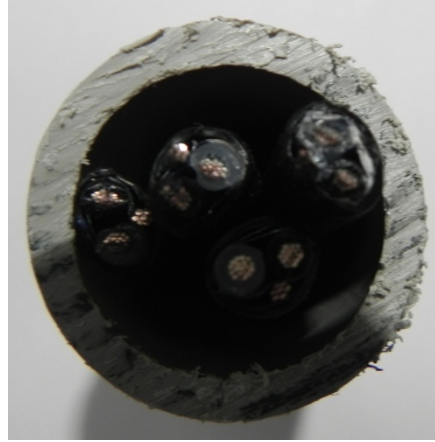
1" conduit w/4 loop feeder cables Exceeds NEC max fill Exceeds ODOT max fill
