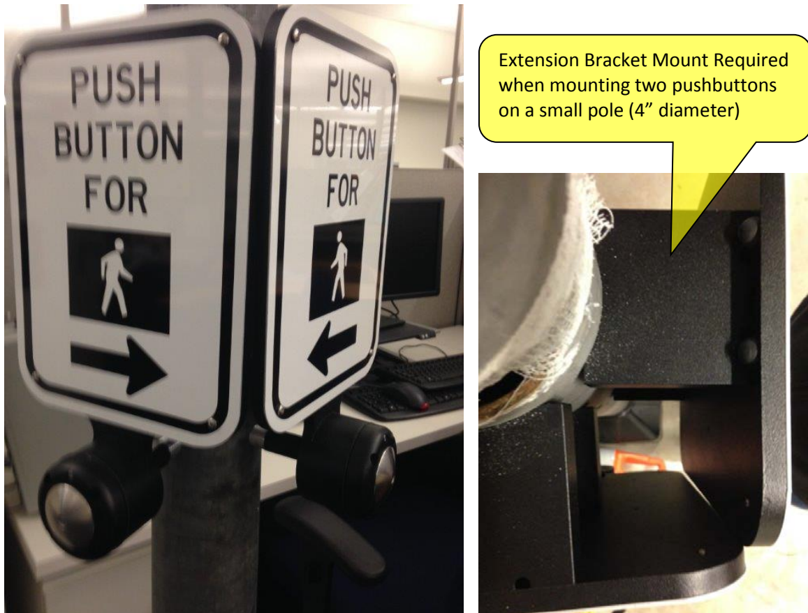
Figure 5-74 | Extension Bracket Mount for Two Pushbuttons on 4 Inch Diameter Pole
