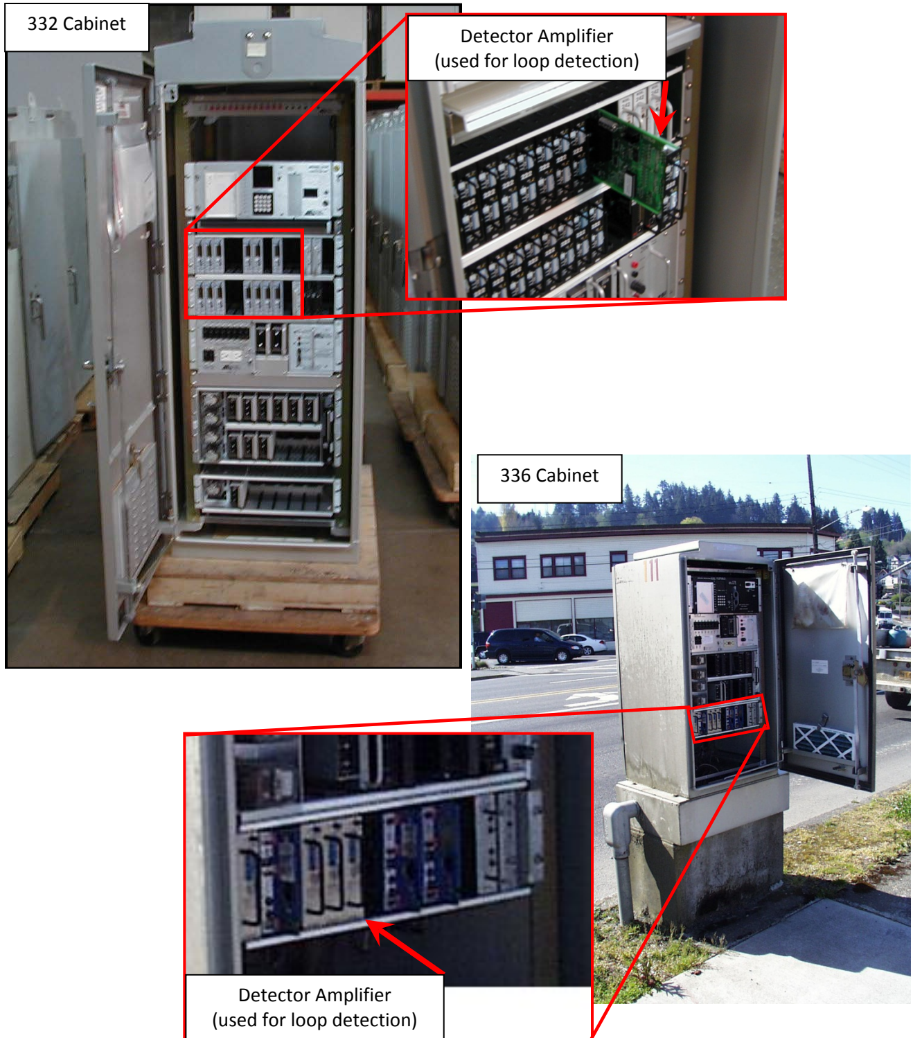
Figure 6-10 | 332 and 336 Signal Controller Cabinet Detection Input File Location
