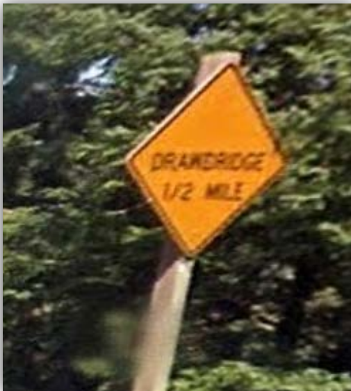
Figure 23-7 | Non-Compliant Existing TCD: Outdated Signs, Example 2
