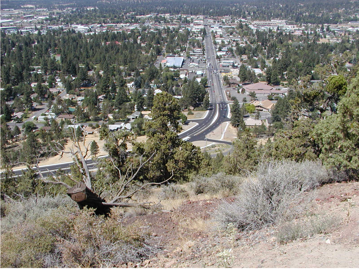
Figure 3.2: View from Pilot Butte of a portion of the U.S. Route 20 project for which a monitoring plan was developed. Stormwater detention basins appear in the center left of the photo.
