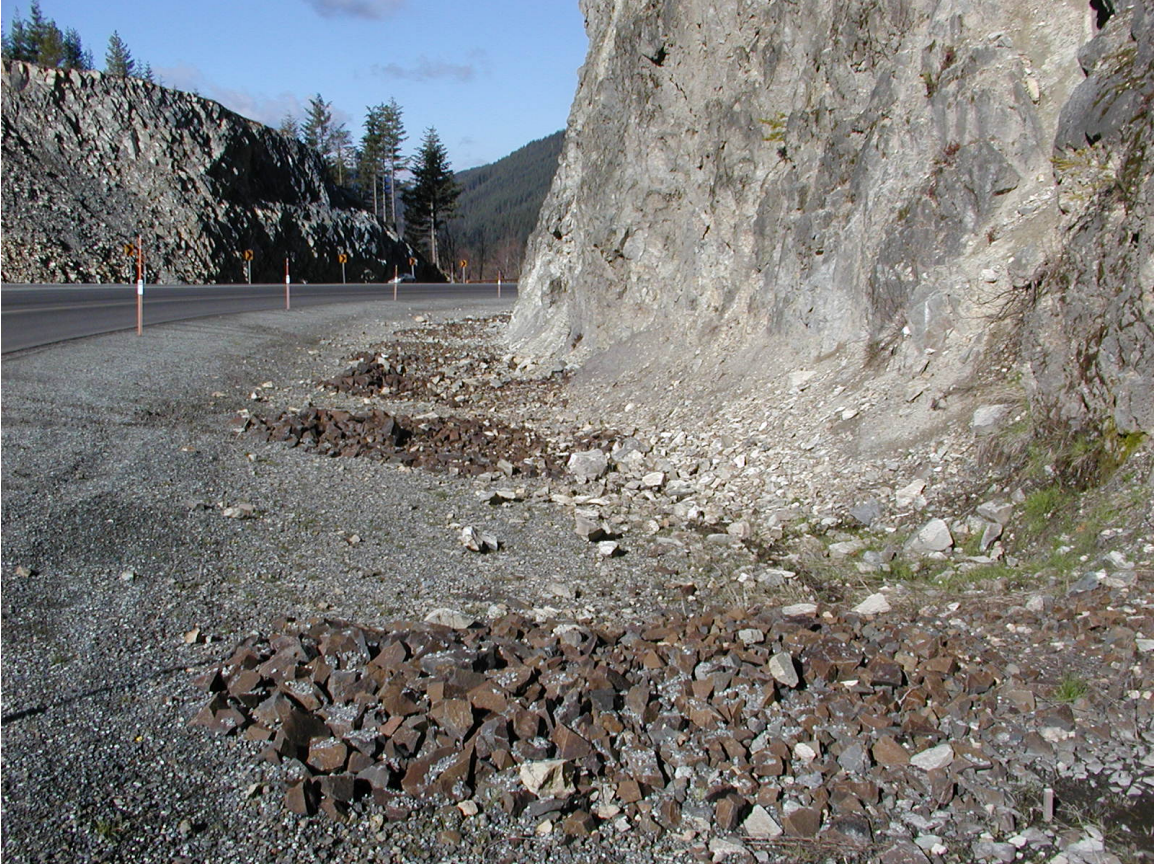
Figure 3.1: View of check dams along U.S. Route 26 at milepoint 49.
