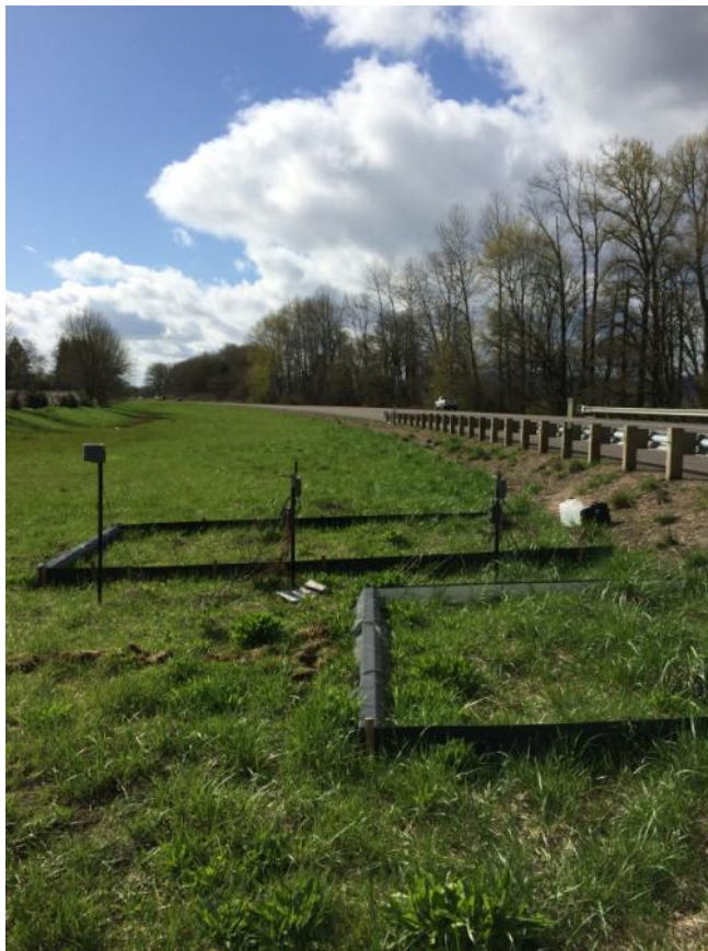
Figure 2.6: Willamette site, southwest view (US Highway 20).
