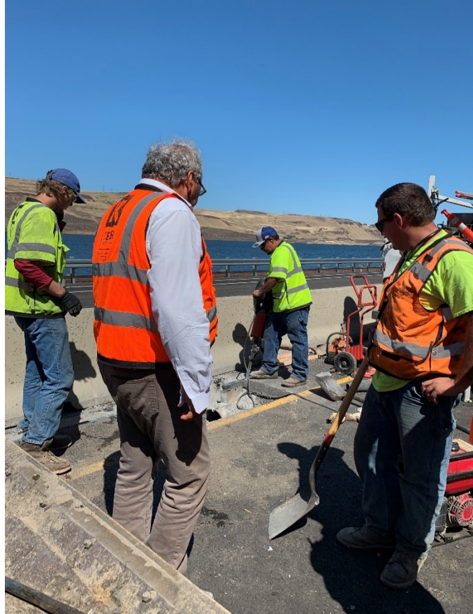
Figure 5.9: Workers on the site (Case study #1)
