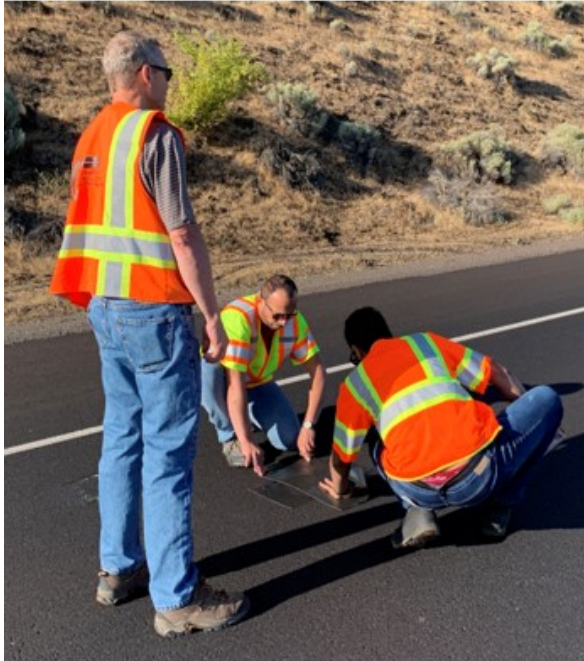
a). Sensor Installation
