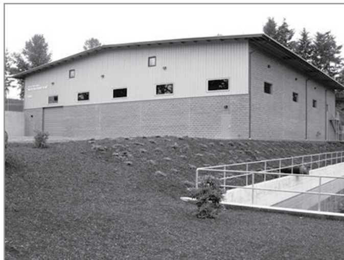
The new WTP in Sweet Home completed in August 2009.
