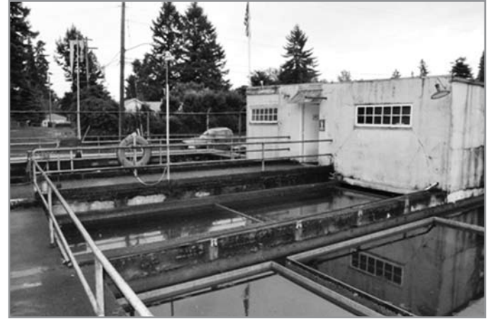
Sweet Home's old treatment facility.
