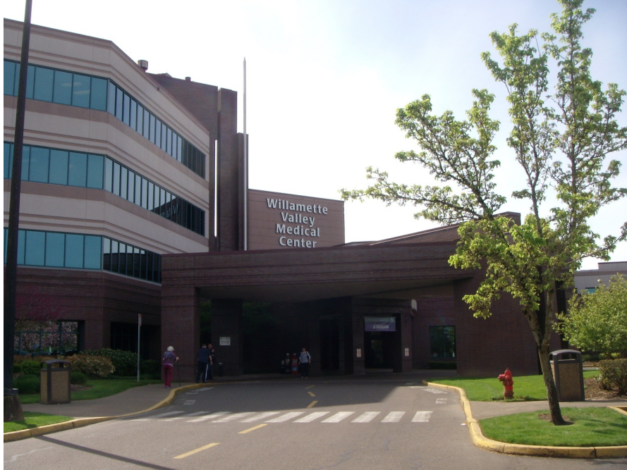
Figure 19. The one-story front entrance of McMinnville hospital (Willamette Valley Medical Center) is next to a four-story building (on the left).
