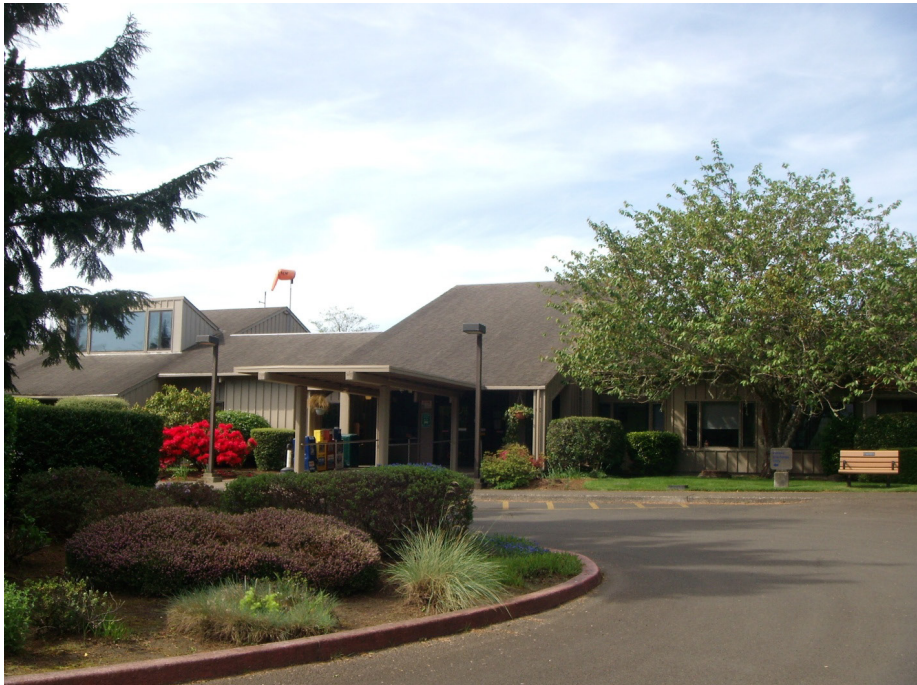
Figure 14. Lincoln City (Samaritan North Lincoln) hospital. Front entrance.
