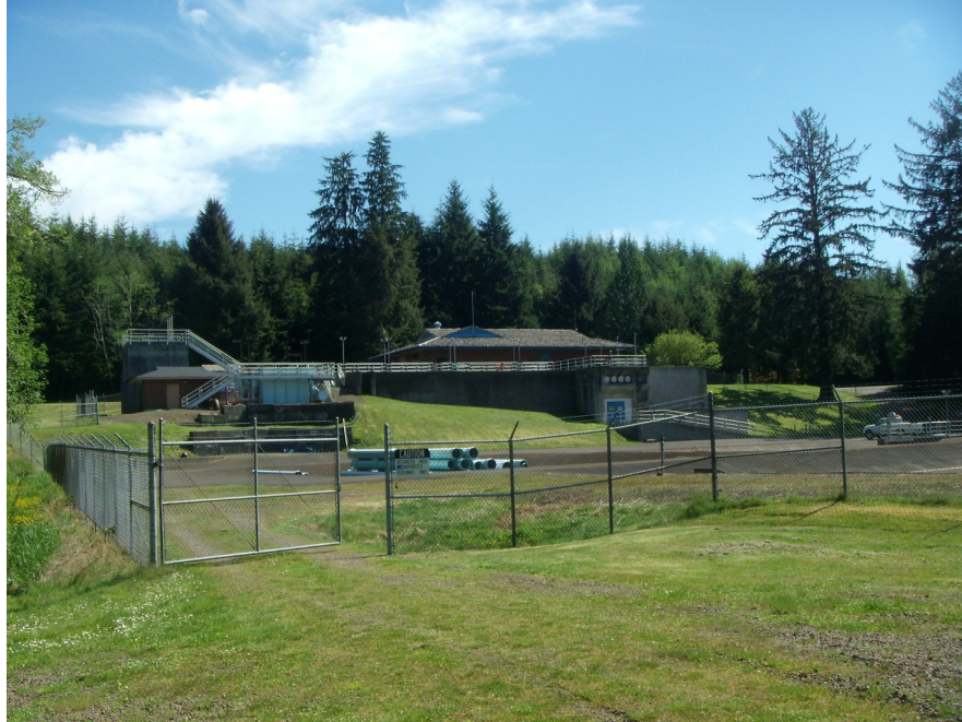
Figure 21. City of Lincoln City Water Treatment Plant, which is a critically important facility and part of the water system that serves the local hospital.
