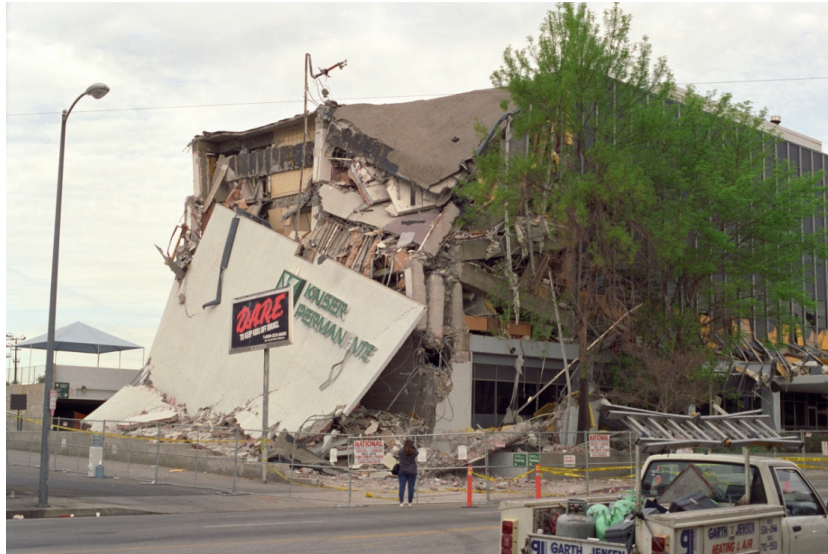
Figure 4. Damage to a Kaiser Permanente hospital in the 1994 magnitude 6.7 Northridge, California earthquake. (Photo by Gary B. Edstrom, http://en.wikipedia.org/wiki/1994_Northridge_earthquake#mediaviewer/File:Kaiser Permanente Building After Northridge Earthquake.jpg )
