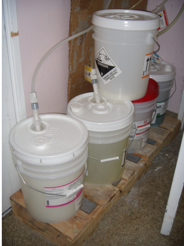
Figure 18. Lincoln City (Samaritan North Lincoln) hospital has potentially hazardous chemicals that are not secured to withstand earthquake shaking and may spill.
