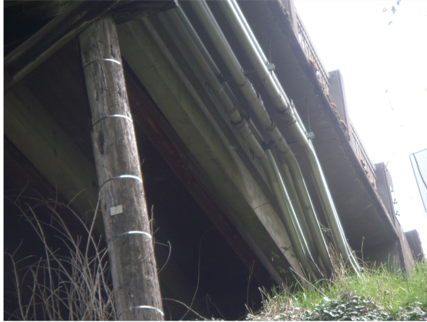
Figure 32. Close-up of the south abutment of Three Mile Lane bridge showing colocated lifelines, including a major telecommunication line. Earthquake-induced bridge damage could disrupt communication services.
