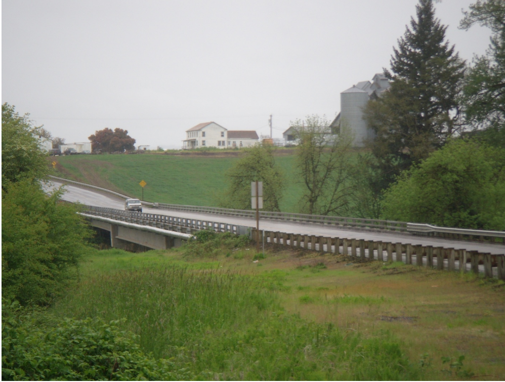
Figure 44. The new bridge on SE Lafayette Highway may be a viable emergency detour for McMinnville residents needing to cross the Yamhill River to access the hospital assuming the bridges in McMinnville are impassable.
