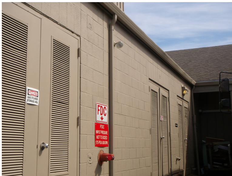
Figure 15. Lincoln City (Samaritan North Lincoln) hospital structure with boilers and mechanical equipment necessary for hospital operations.
