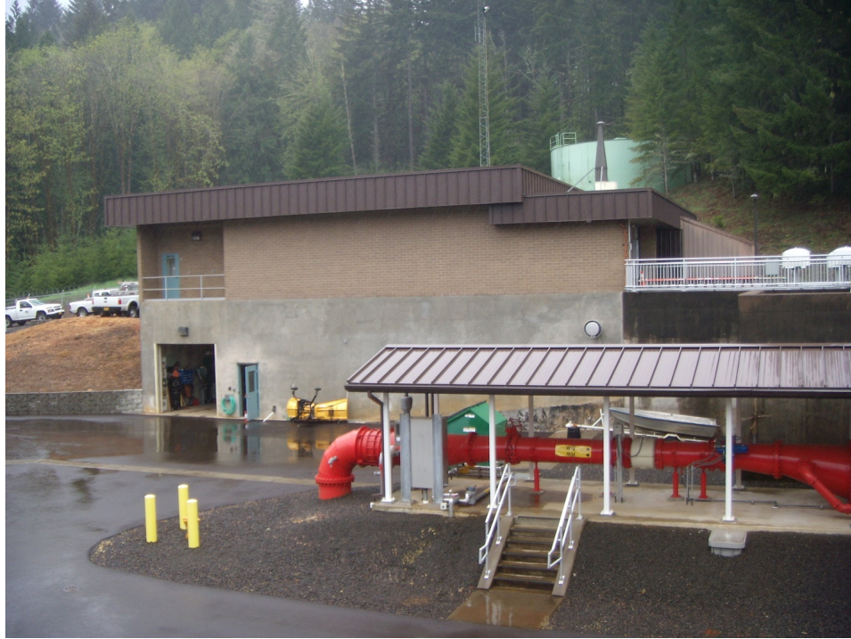
Figure 23. McMinnville Water and Light Water Treatment Plant showing the control building. This is a critically important facility that serves the local hospital.
