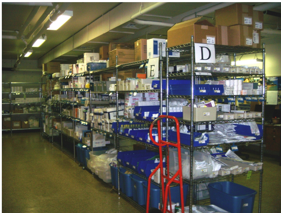
Figure 17. Lincoln City (Samaritan North Lincoln) hospital with contents damage potential, such as medical supplies falling off the shelves that have not been seismically secured.
