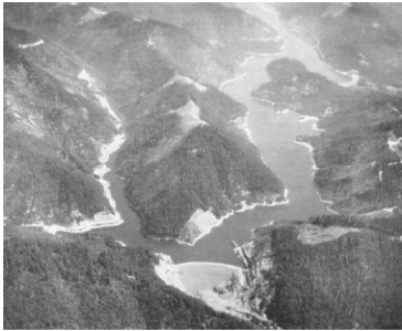
Source: Oregon National Guard, 1981-82. View looking northeast.
