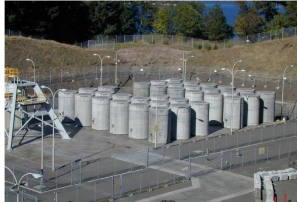
Concrete and steel storage canisters at the former Trojan site.
