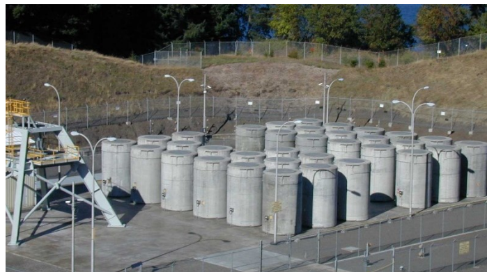
Figure 2. ISFSI Transfer Station (left) and Storage Casks (right)
