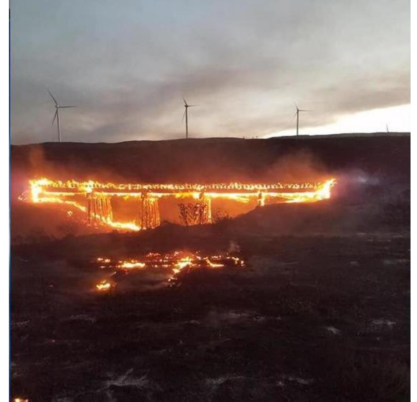
Photo Credit: North Gilliam Fire Protection District. Source: https://katu.com/news/local/wind-turbine-sparks-fire-in-arlington
