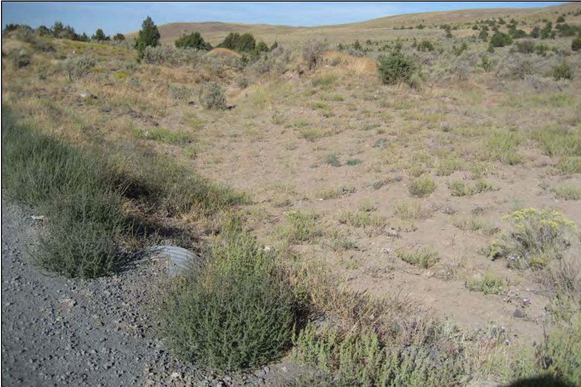
Photo Plate 6 View northeast showing drainage S27, China Ditch. Existing gravel access road crosses drainage with a 24-inch culvert (9/12/2006).
