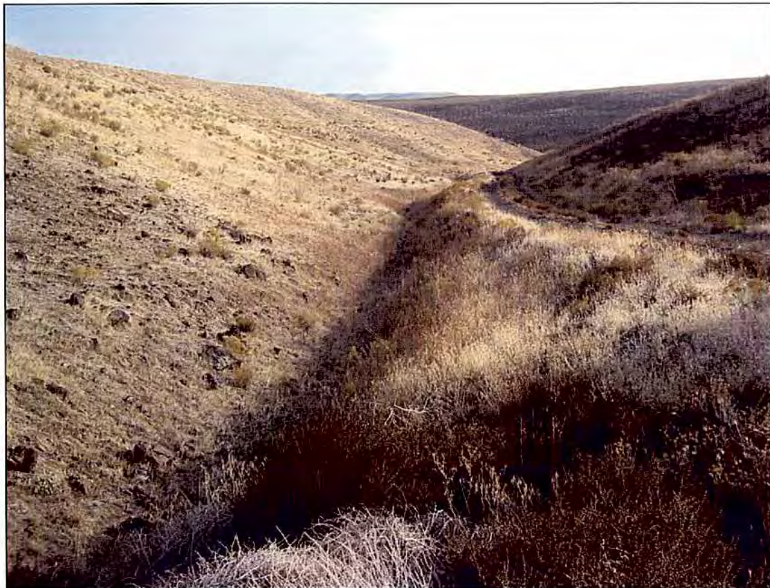
Photo Plate 24 View southeast showing drainage channel adjacent to roadway at S20.
