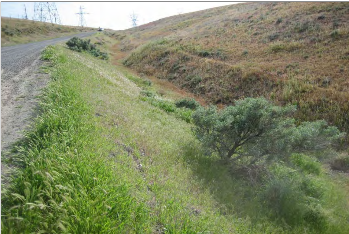
Photo Plate 4 View northeast showing drainage S25. Mostly vegetated at this location, bed and banks and evidence of flow become more defined downstream. Channel drains to China Creek (5/5/2006).
