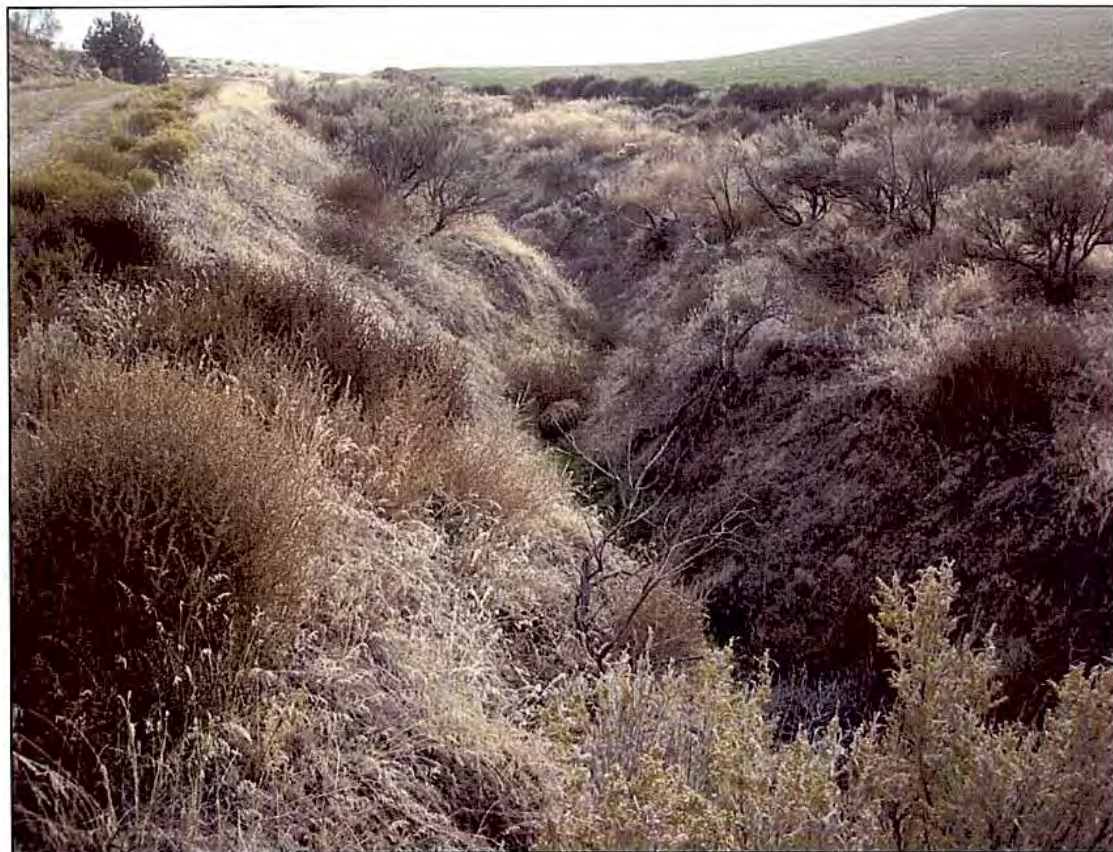
Photo Plate 8 View south showing drainage channel adjacent to roadway at S7.
