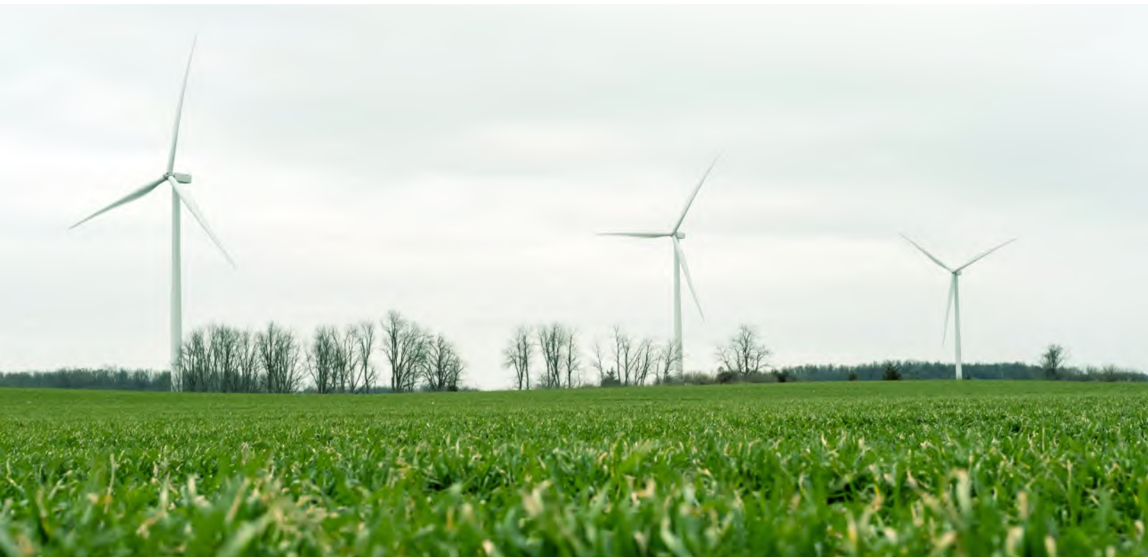
The 119-megawatt Bluff Point Wind Energy Center in Indiana.
