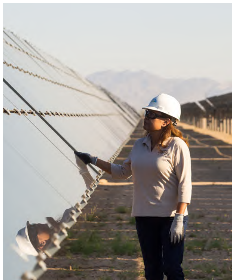
A solar technician inspects the panels at the Blythe and McCoy Solar Energy Centers in California.
