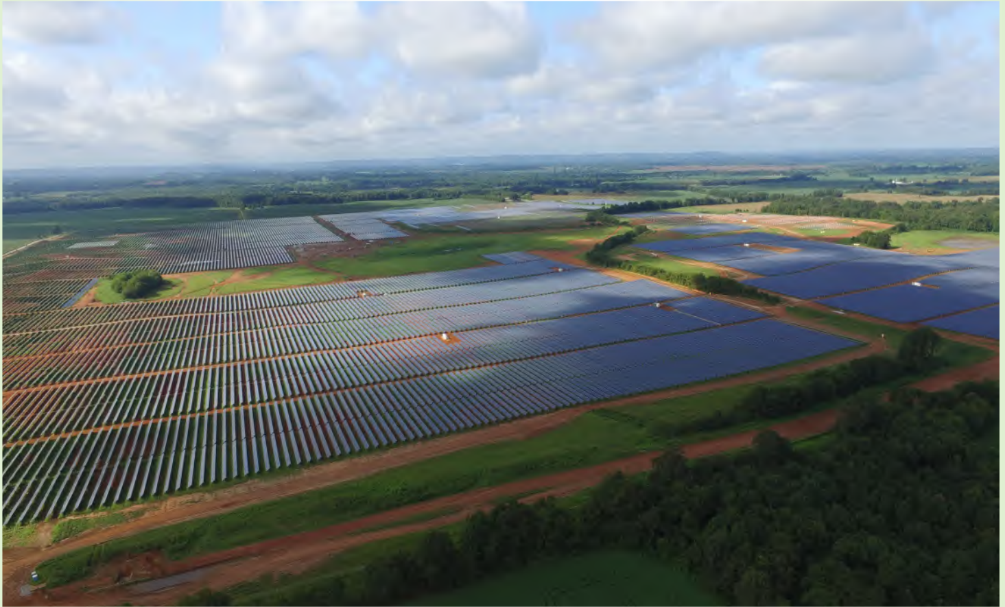
The 75-megawatt River Bend Solar Energy Center in Alabama.
