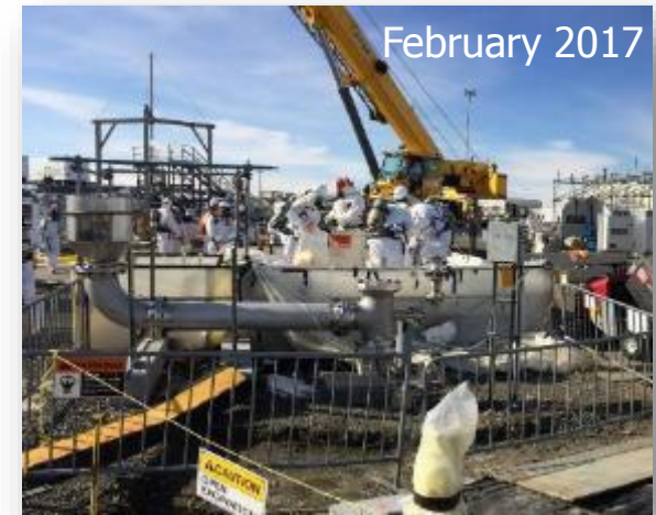
C-105 retrieval operations completed in November 2017
