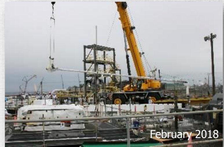
Pump removal from AX-102
