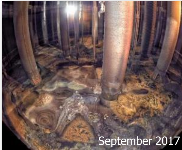
AY-102 interior after retrieval
