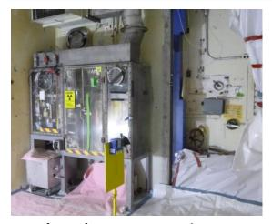
Workers began removing a glovebox at the 324 Building to support installation of remotely operated equipment.
