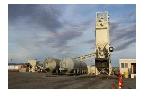
To mitigate traffic effects, workers constructed safeaccess roads and a grout batch plant.
