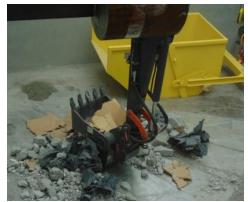
Crews at the 324 Building mock-up installed and tested the first remotely operated excavator.
