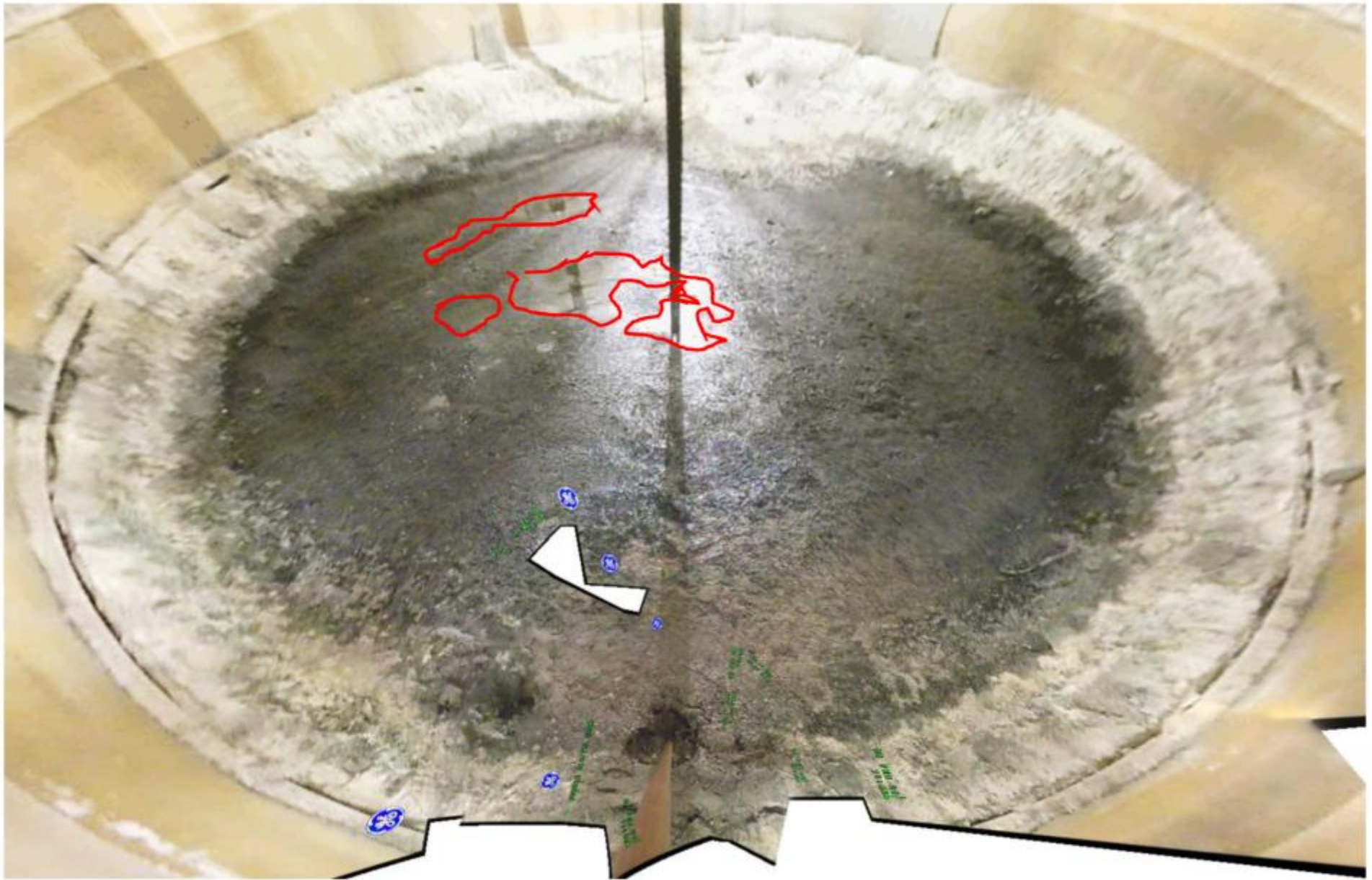
Figure 5-8. Tank B-109 February 5, 2021 Waste Surface Composite View from Riser 7
