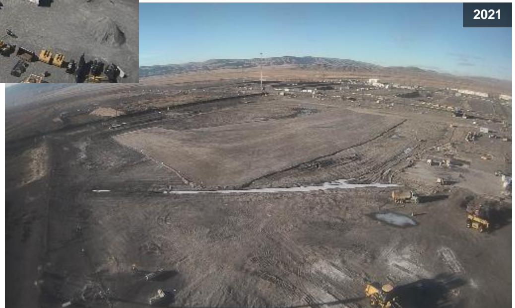
Plutonium Finishing Plant after demolition
