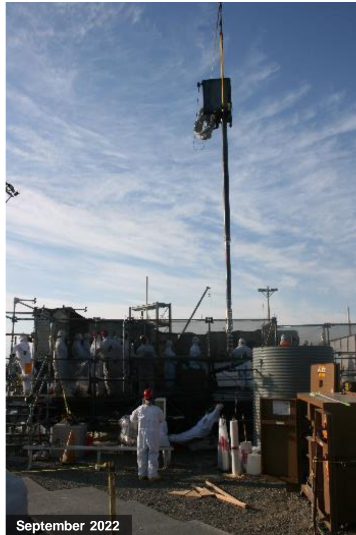
Tank AX-101 A-Pit Riser 5B slurry pump installation
