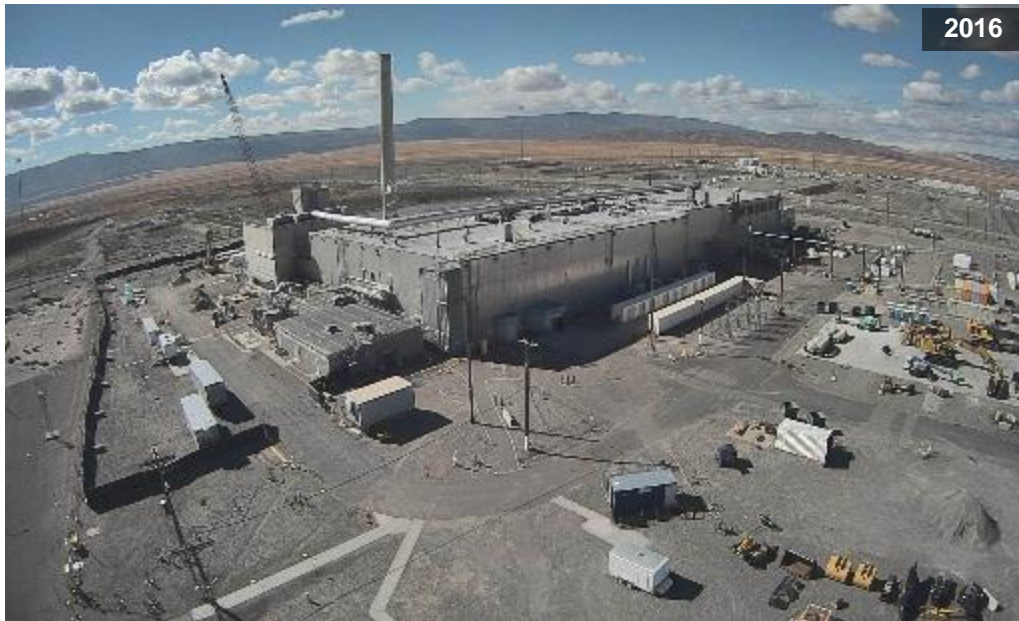
Plutonium Finishing Plant before demolition
