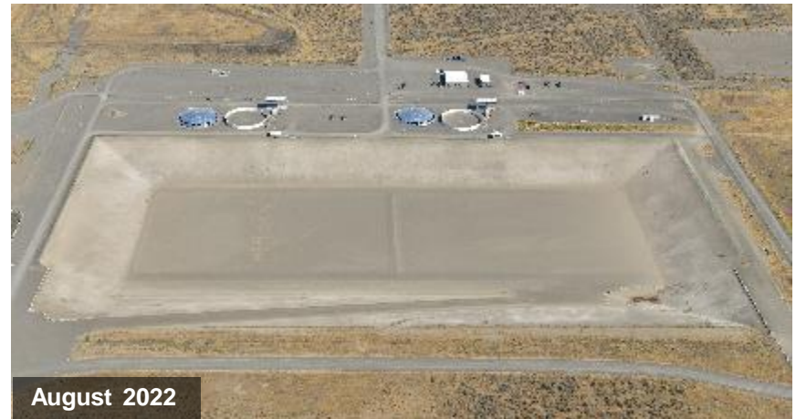
Integrated Disposal Facility
