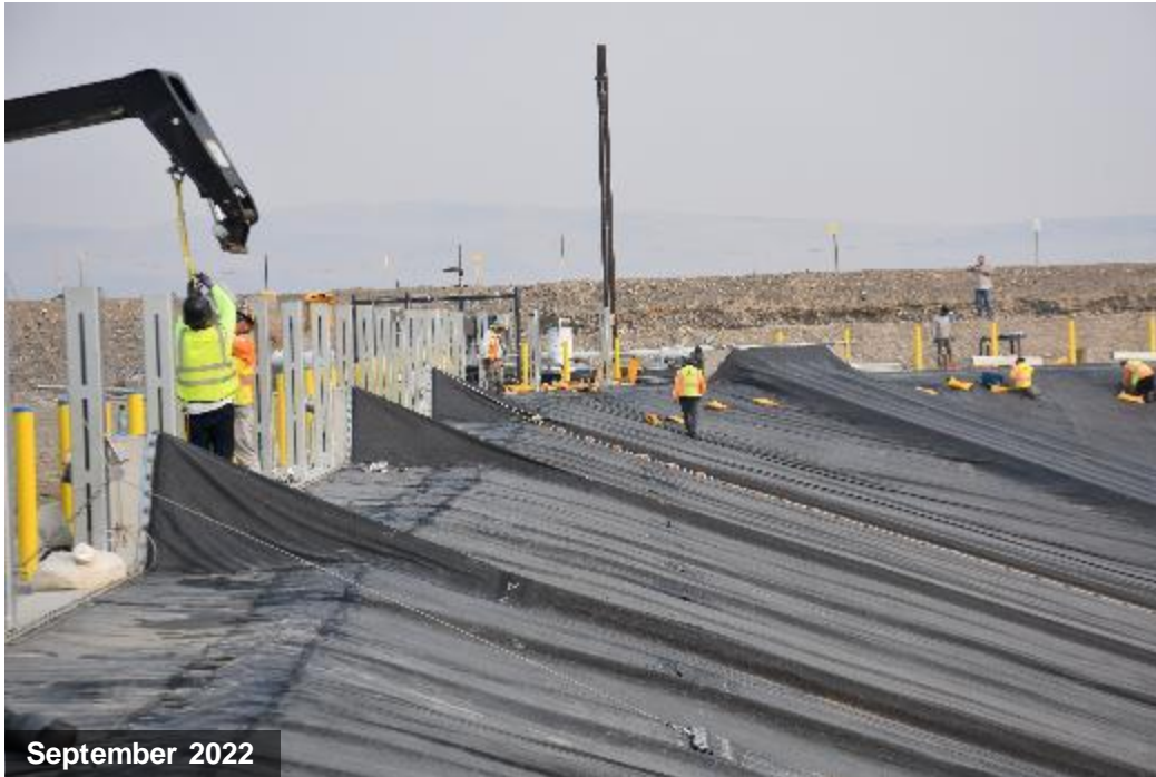
Floating cover installation on wastewater storage basin at the facility
