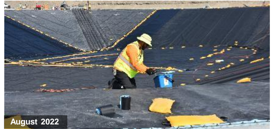
Work progresses at Liquid Effluent Retention Facility Basin 41
