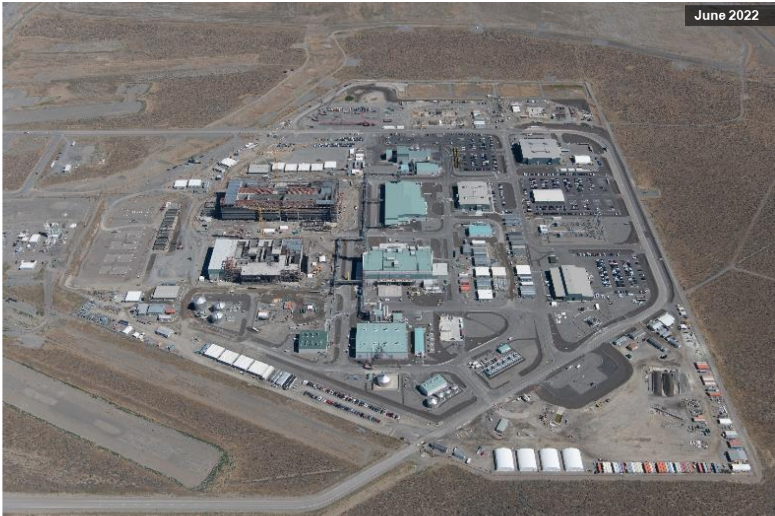
Waste Treatment and Immobilization Plant complex
