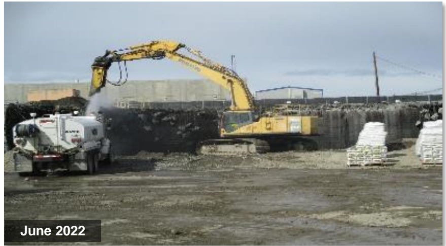
Demolition of K West fuel storage bunker
