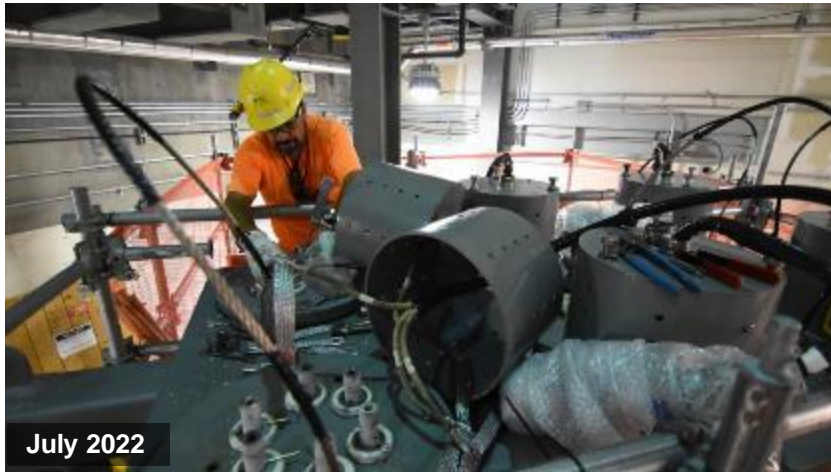
Installing temporary heaters for the startup of Melter 1
