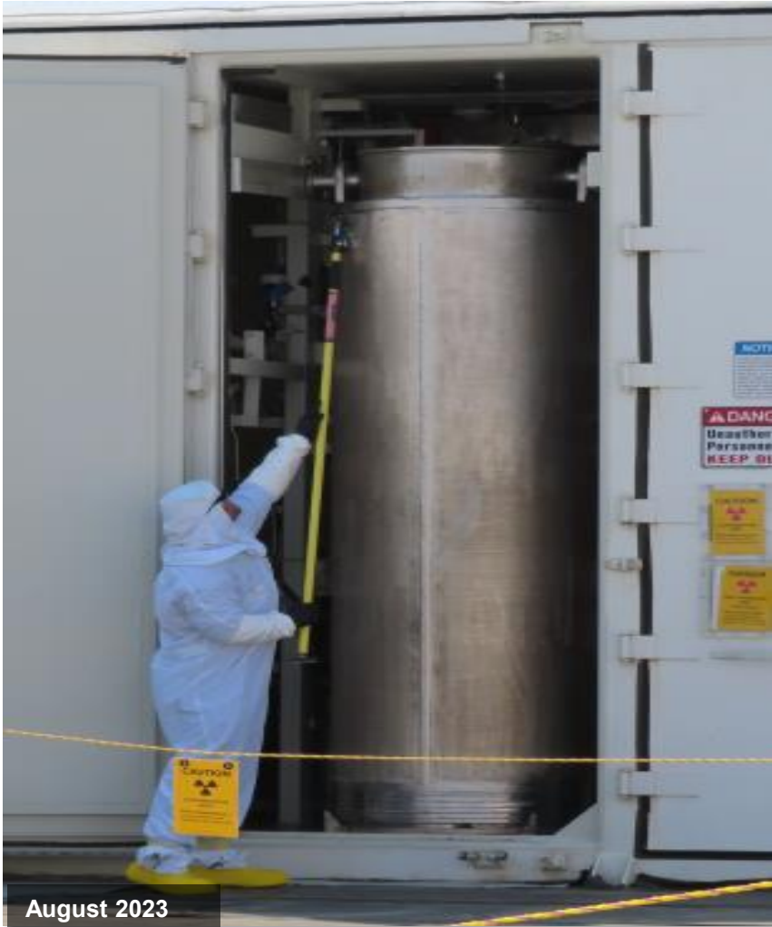
Worker disconnecting ion exchange column in the TSCR System process enclosure
