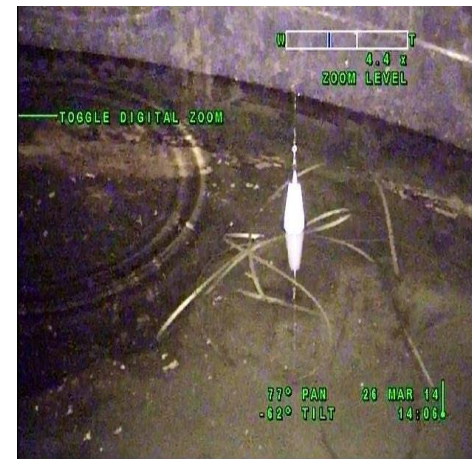
Liquid level measurement
