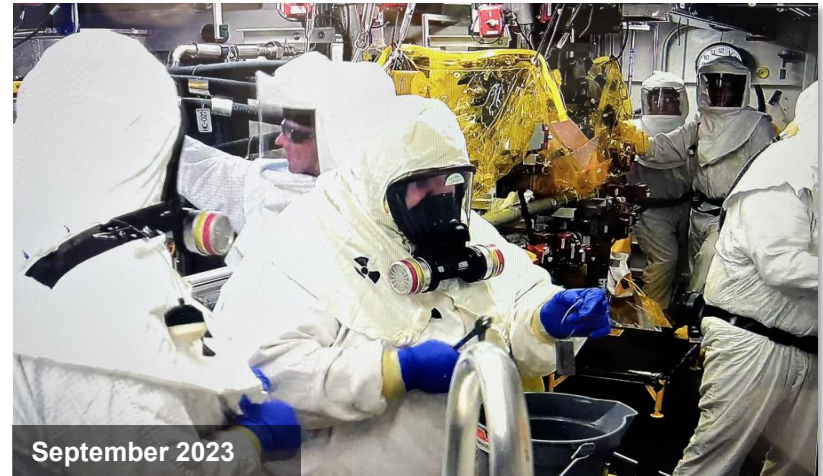
Workers connecting Ion Exchange columns for batch 4 start-up
