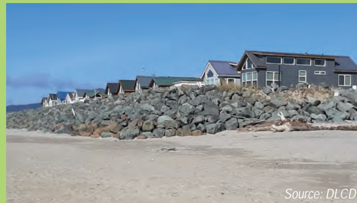
Rip rap in front of homes in Rockaway Beach
