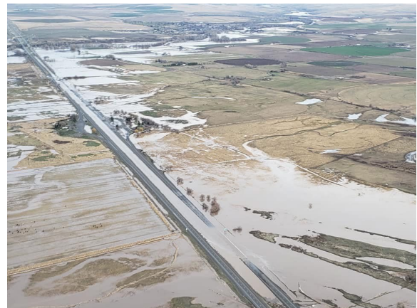
DLCD helps communities plan for and mitigate risks from natural hazards. Umatilla River, 2020. Source: DLCD
