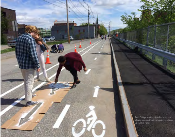
Demonstration buffered two-way bicycle lane.
