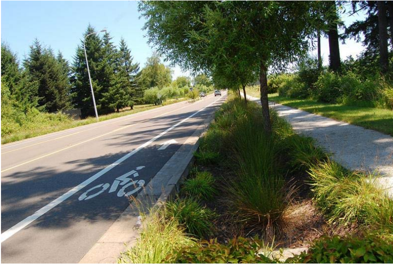
Bike lane, landscape/stormwater, permeable sidewalk
