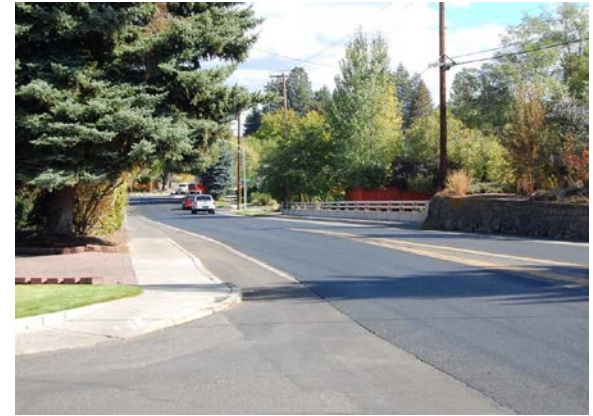
Sidewalks on bridge
