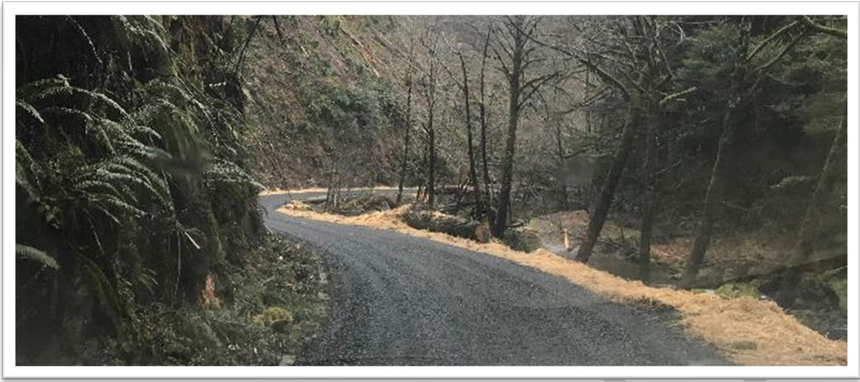
Photo 3. Example of other measures, mulching.
