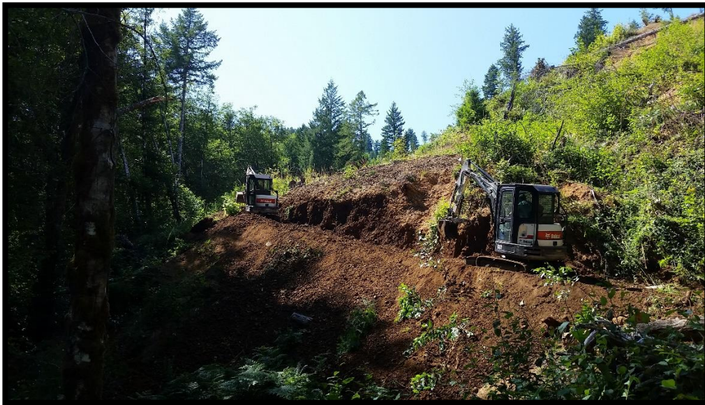
Mongo's Trail re-construction due to landslide-TSF
