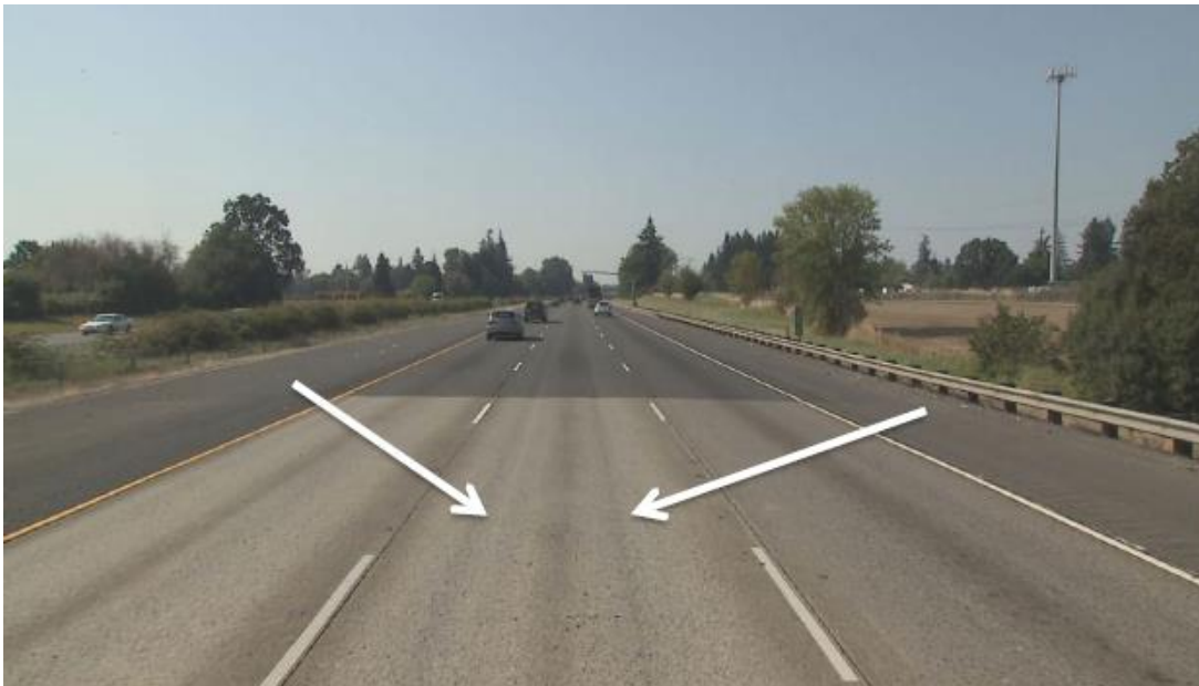
I-5 SB segment near Wilsonville showing wheel rut wear caused by studded tires (Shippen, Kennedy et al. 2015)
