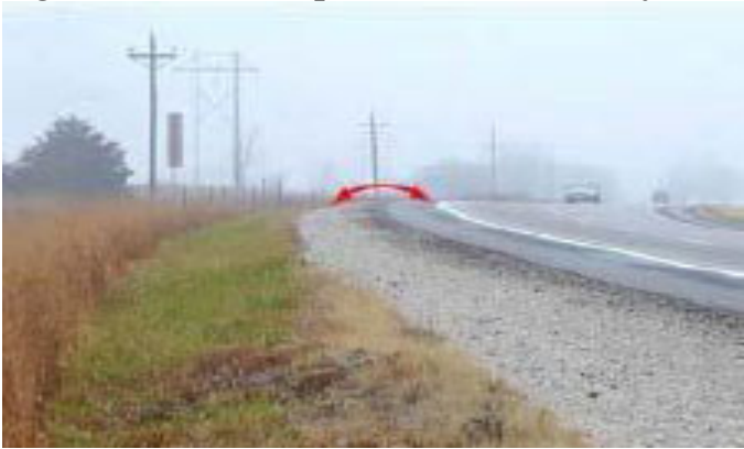
Figure 6-3. Side Slope on Rural Roadway
