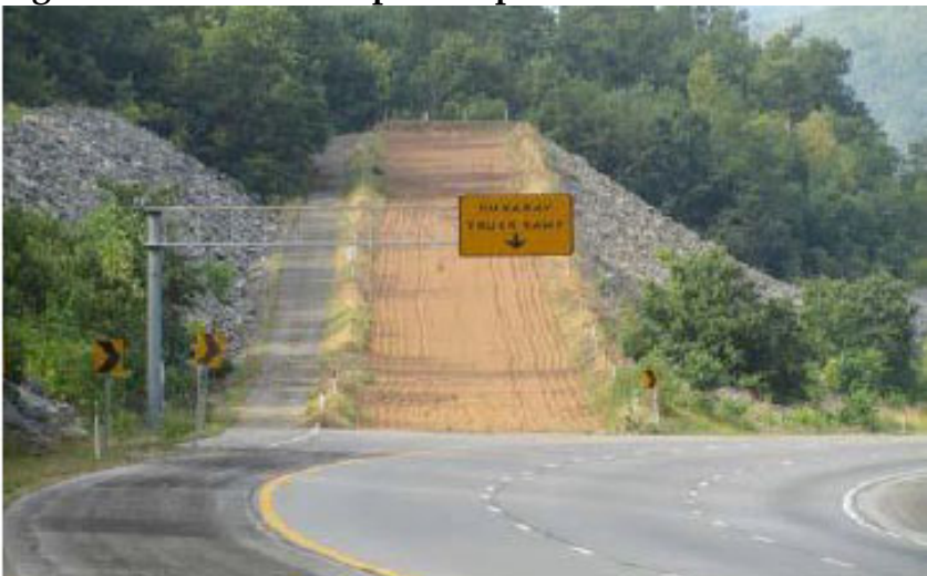
Figure 3-54. Truck Escape Ramp
