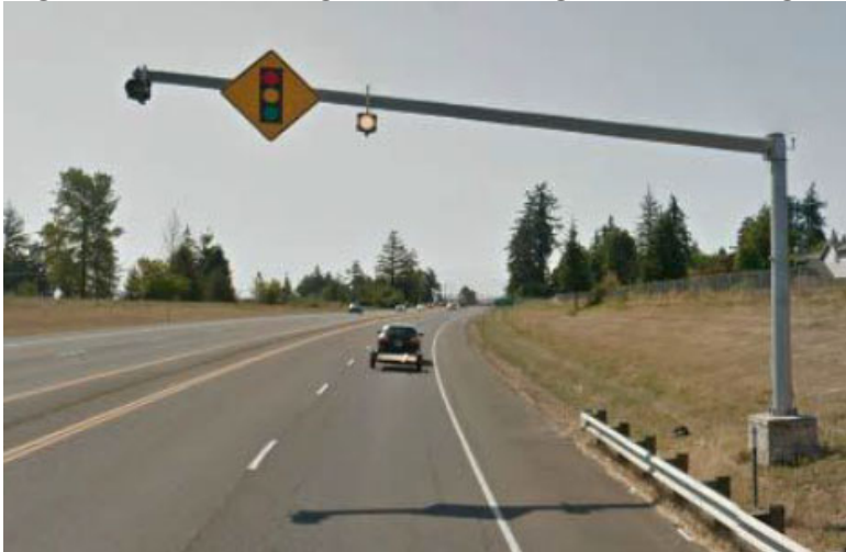
Figure 4-15. Flashing Beacon on Signal Ahead Sign
