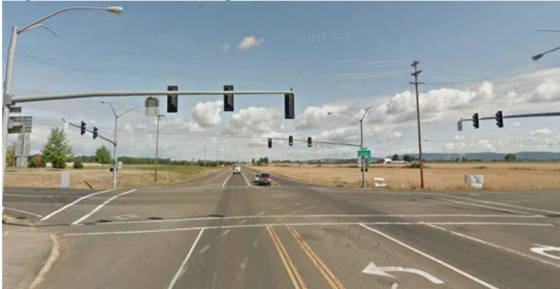
Figure 3-24. Traffic Signal at Rural Intersection
