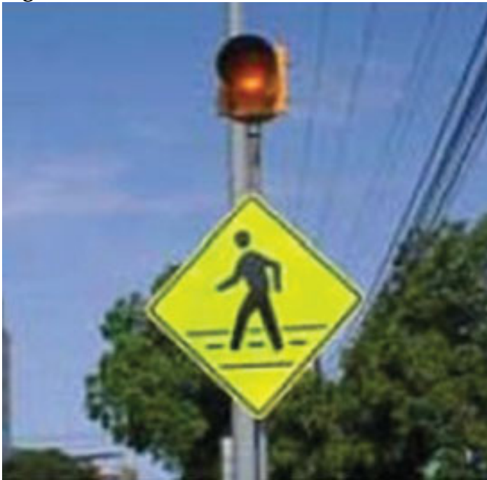
Figure 5-12. Pedestrian Activated Beacon
