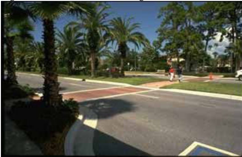
Figure 5-13. Pedestrian Crossing at Midblock
