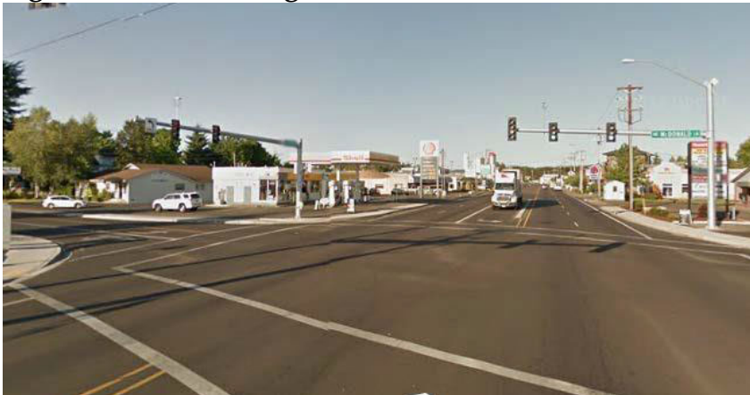
Figure 3-22. Traffic Signal at Urban Intersection
