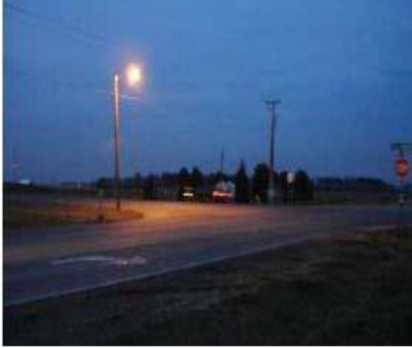
Figure 3-29. Lighting at Intersection
