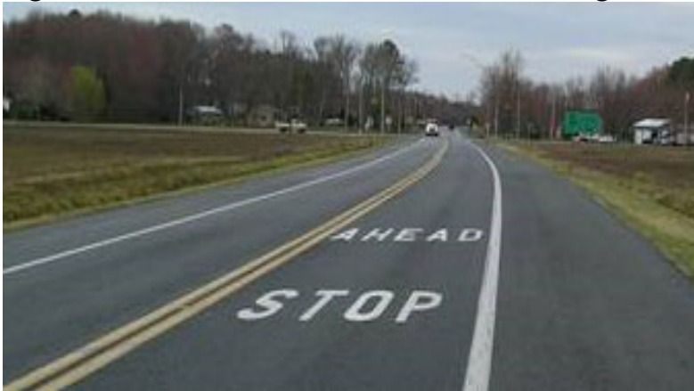
Figure 4-30. STOP AHEAD Pavement Marking
