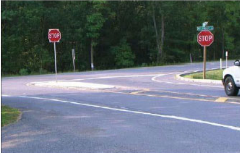
Figure 4-28. Splitter Island at Stop-controlled Intersection
