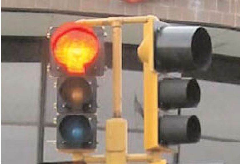
Figure 4-4. Signal Heads with 8-inch and 12-inch Lens
