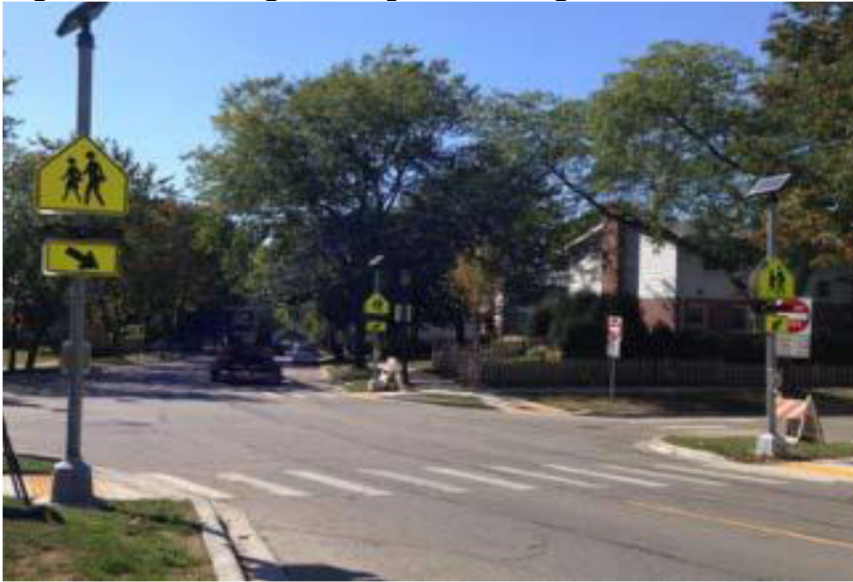
Figure 5-9. Rectangular Rapid Flashing Beacon
