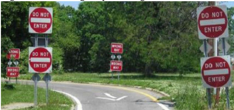
Figure 4-32. Wrong Way Driving Countermeasures
