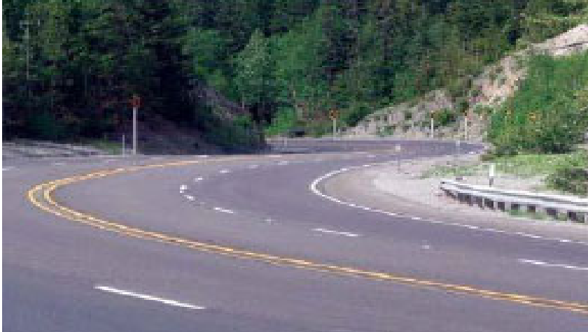
Figure 3-43. Flatten Horizontal Curve on Roadway Segment
