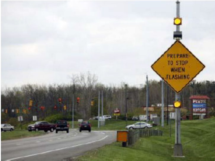
Figure 4-16. Flashing Beacon for Signalized Intersection
