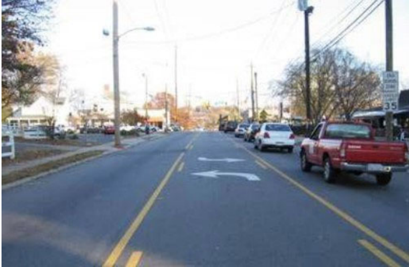
Figure 3-33. Two-way Left-turn Lane
