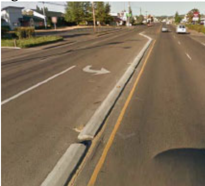
Figure 3-17. Left Turn Channelization with Raised Median
