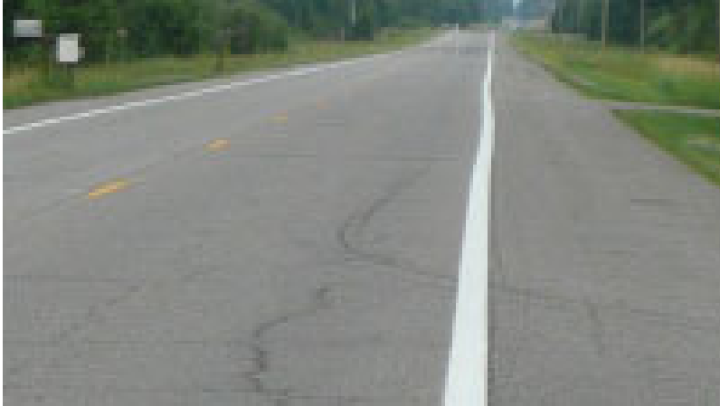
Figure 6-24. Wide Edgeline for Roadway Segment
