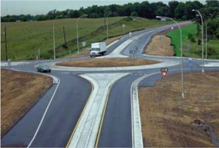
Figure 3-18. Roundabout at Unsignalized Intersection
