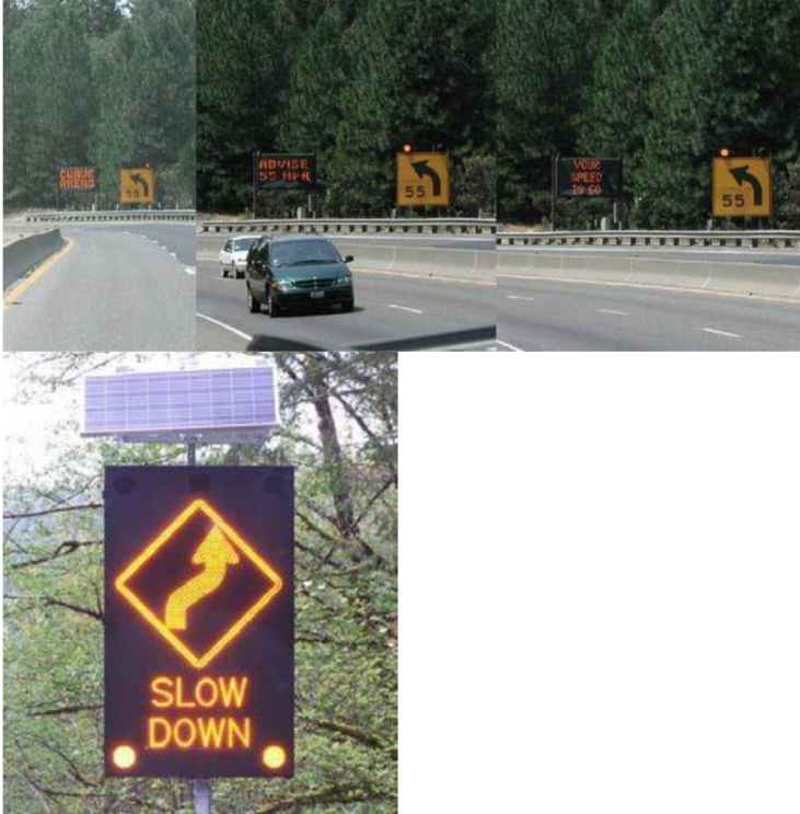
Figure 6-11. Dynamic Speed Feedback Sign for Curve
