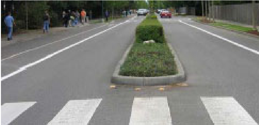
Figure 3-37. Raised Median on Urban 2-lane Road
