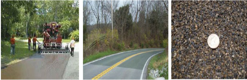
Figure 3-48. High Friction Surface Treatment for Curve Segment
