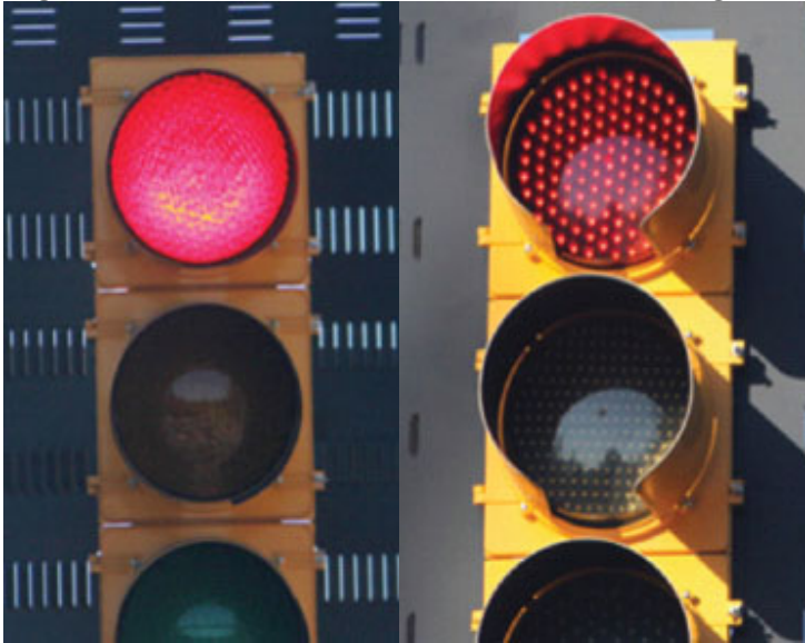
Figure 4-6. Incandescent and LED Traffic Signal Head
