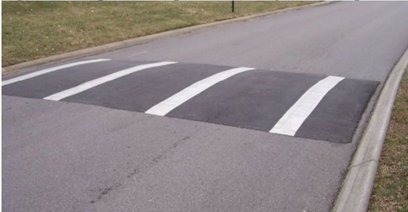
Figure 5-30. Speed Hump for Reducing Vehicle Speed
