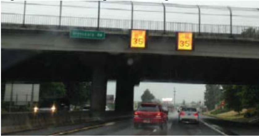
Figure 3-50. Variable Speed Limit Sign
