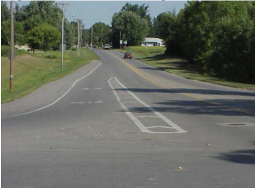
Figure 3-65. Offset Right-turn Lane at Intersection
