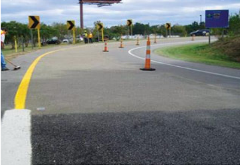
Figure 3-49. High Friction Surface Treatment on Ramp
