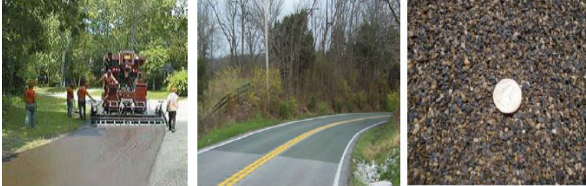
Figure 4-18. High Friction Surface Treatment
