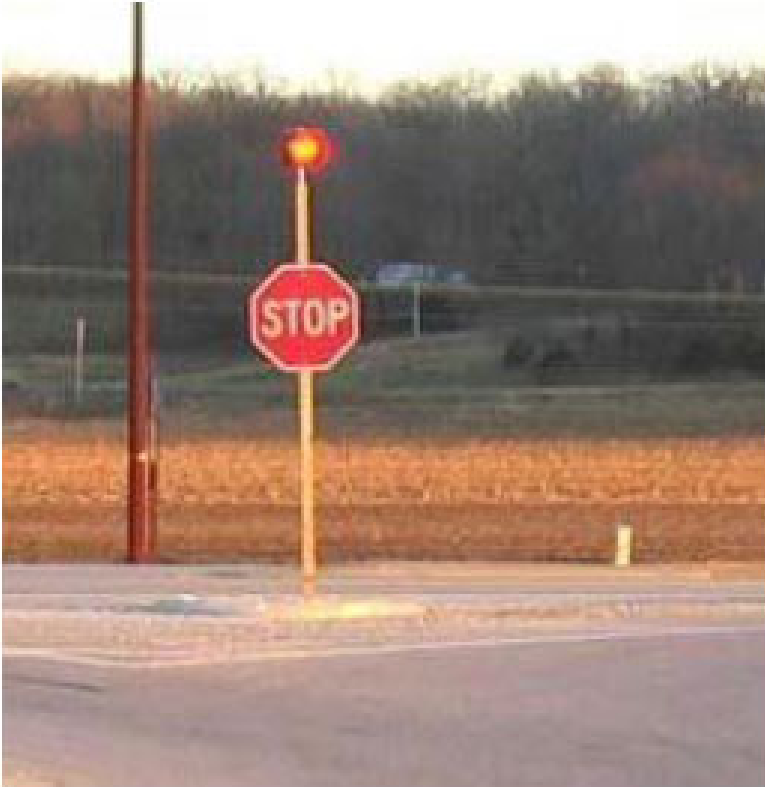
Figure 4-24. Flashing Beacons at All-way Stop Controlled Intersection
