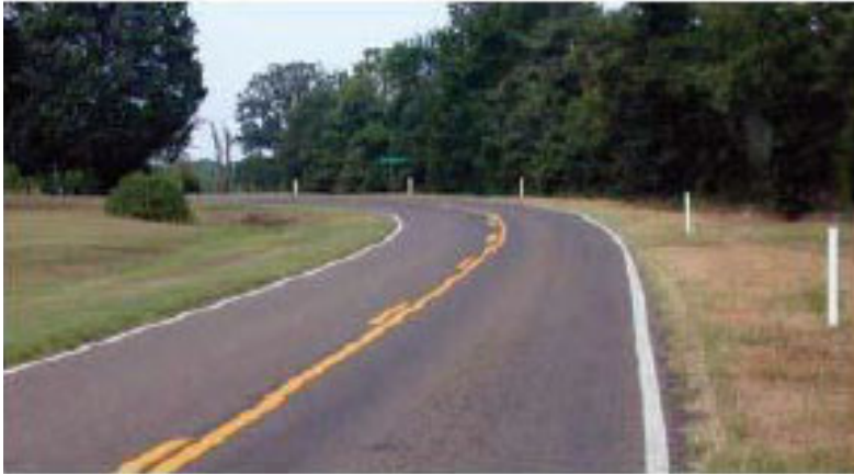
Figure 6-14. Post-mounted Curve Delineator
