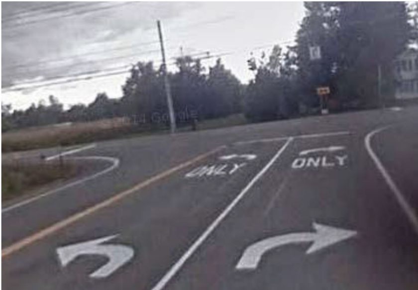
Figure 3-14. Left Turn Channelization at Rural Signalized Intersection
