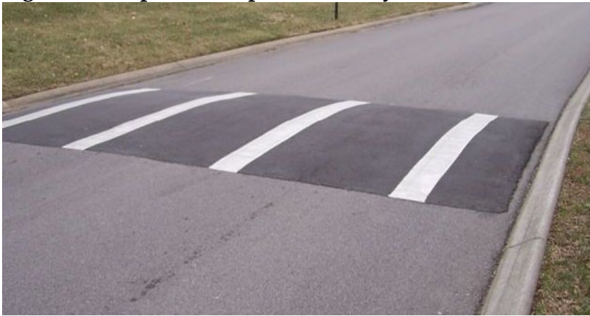
Figure 3-66. Speed Hump on Roadway
