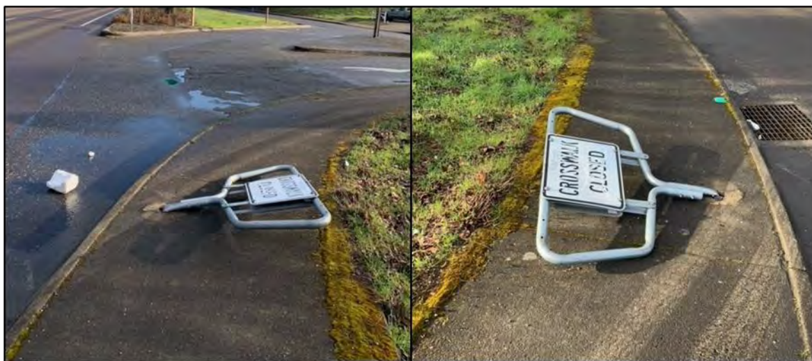
Figure 310.8-1: Damaged Crosswalk Closure Treatment
