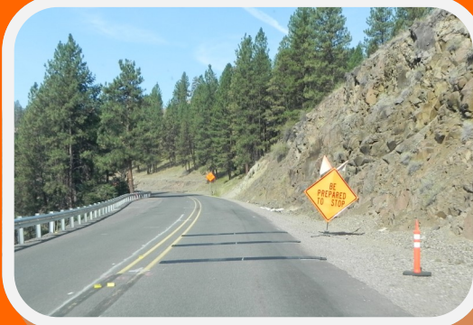
(Above) Portable Rumble Strip use with flagger operation.
