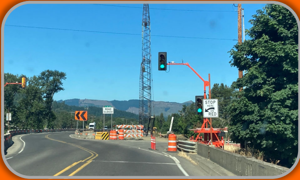
(Below) Temporary Portable Traffic Signal usage during bridge replacement project.
