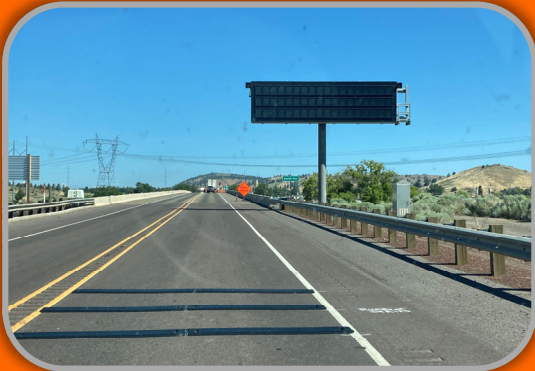
(Above) Portable Rumble Strip use with flagger operation.
