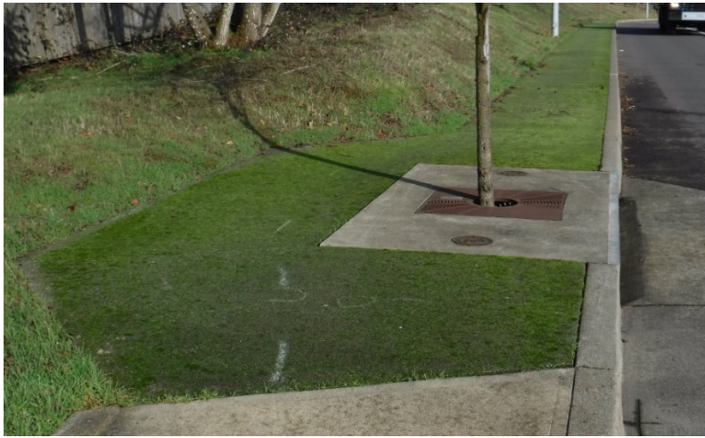
Figure 800-23: Porous Pavement Installed Next to Concrete Walk Illustrating Mossy Growth
