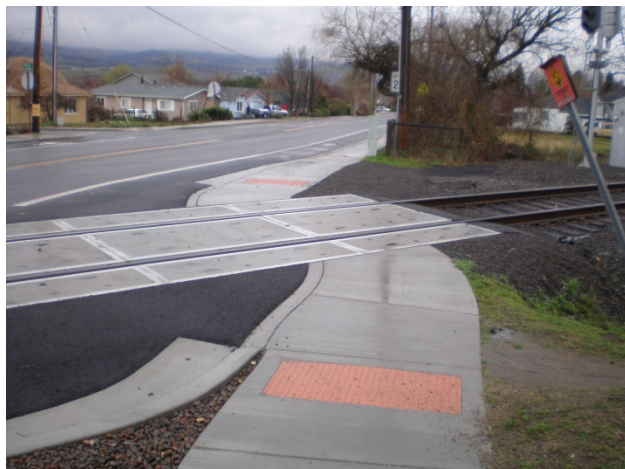
Figure 800-70: Skewed Walkway and Rail Track Crossing
