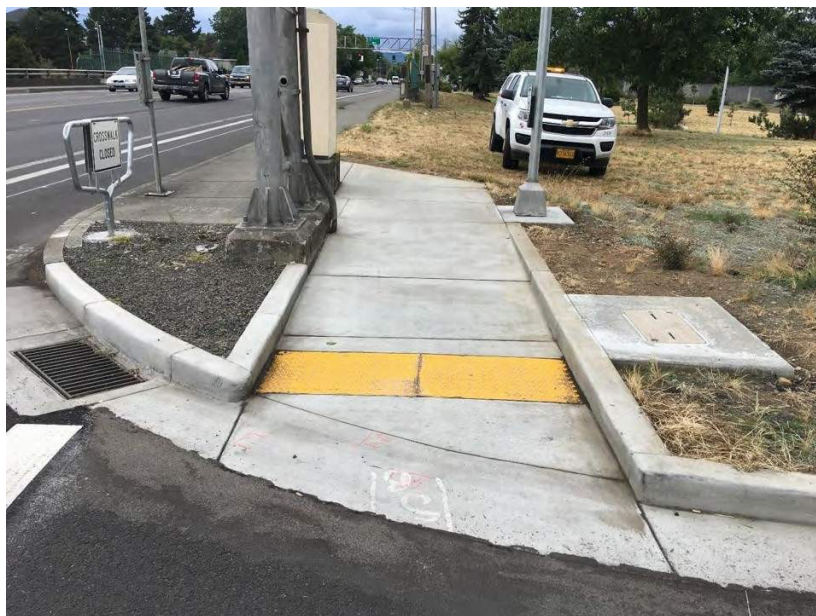
Figure 800-61: Directional Curb with Grade Break Less than 5 feet and No Flare Photo
