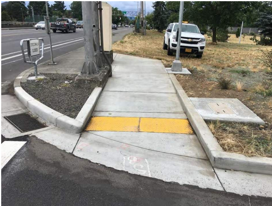
Figure 800-44: Curb Ramp System with a Directional Curb
