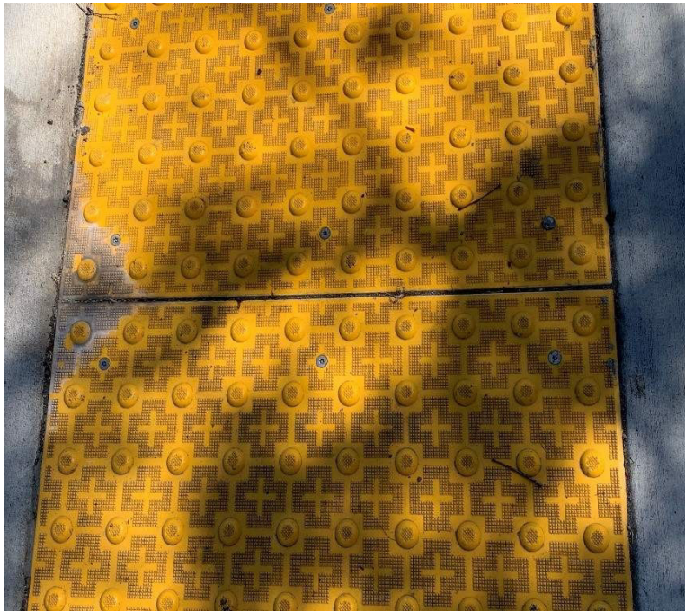
Figure 800-52: Wet Set Polymer Detectable Warning Surface Tile Dome Spacing is Maintained
