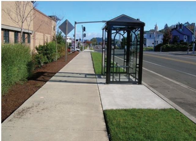
Figure 800-31: Bus Shelter in Buffer Zone
