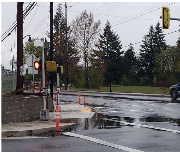
Figure 800-45: Water Accumulation at Curb Ramp on Landing/Turn Space
