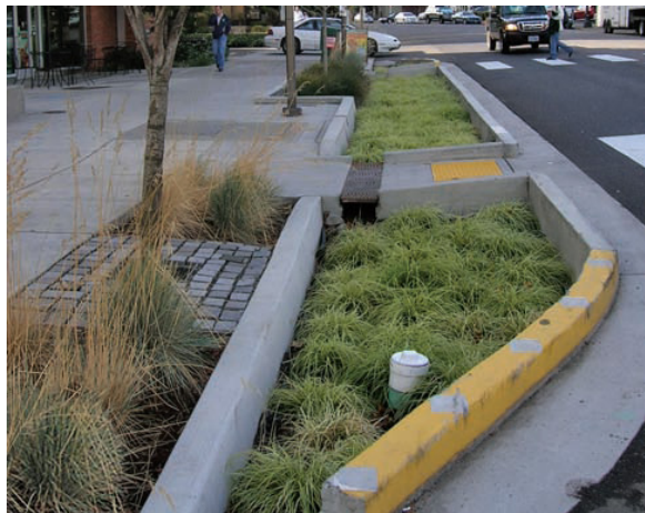
Figure 800-9: Landscaping Providing Storm Water Treatment
