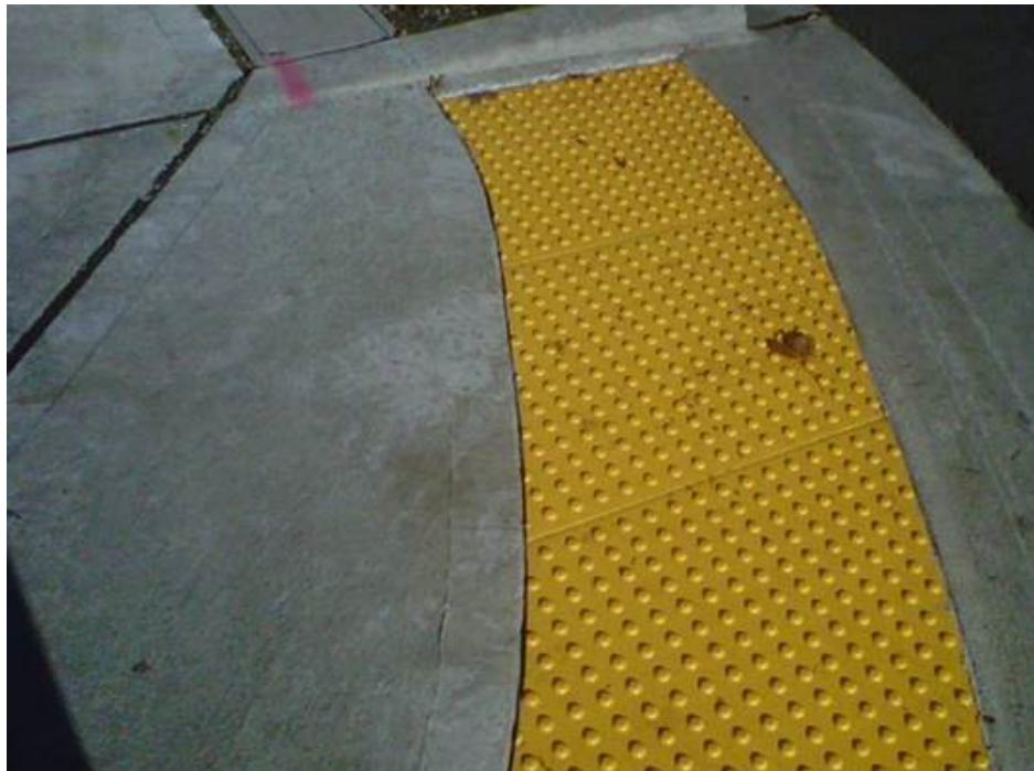
Figure 800-57: Example 2, Detectable Warning Surface Rectangular Tile Cutting to Fit Radius
