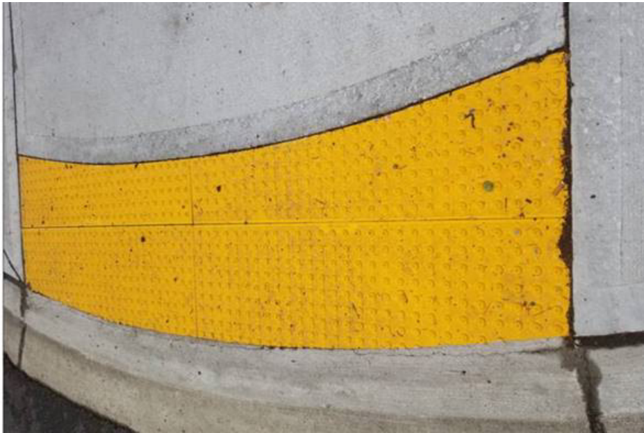
Figure 800-57: Example 2, Detectable Warning Surface Rectangular Tile Cutting to Fit Radius
