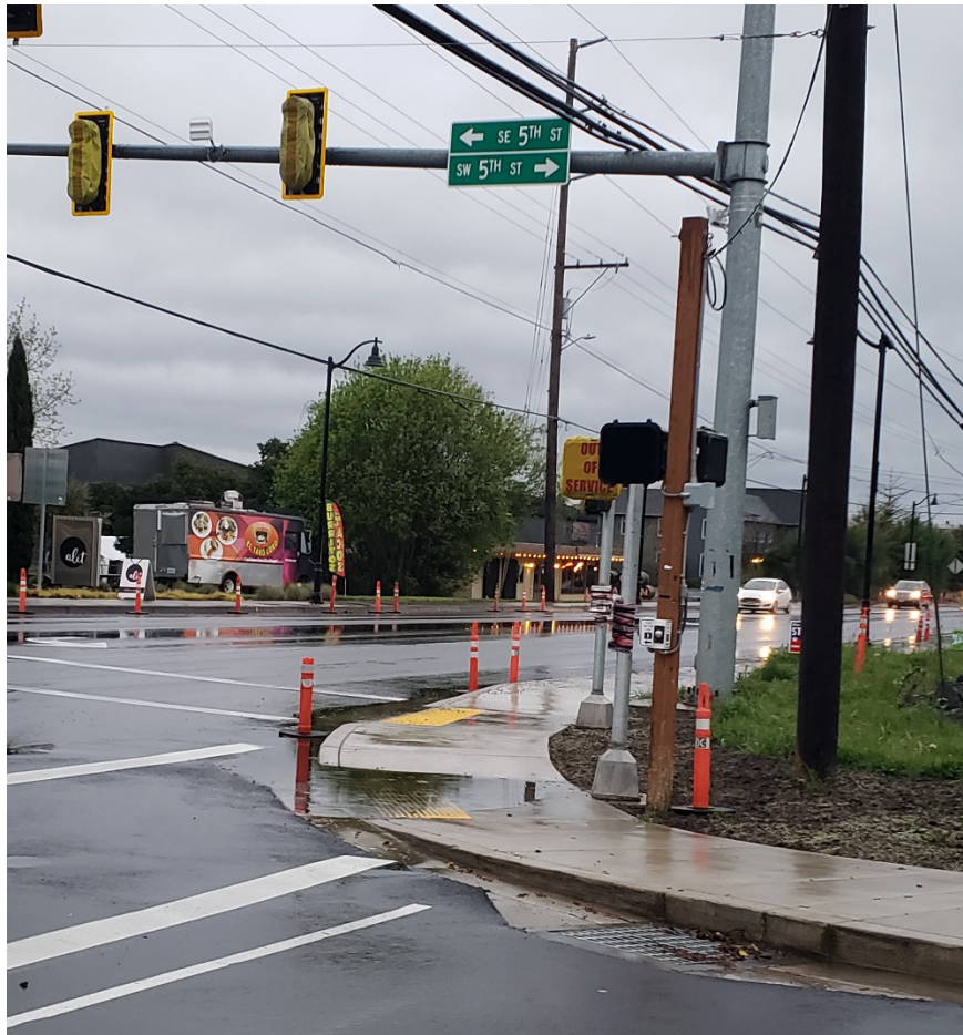
Figure 800-37: Water Accumulation at Curb Ramp
