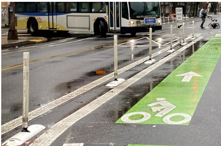
Figure 900-12: Tubular markers as street buffer
