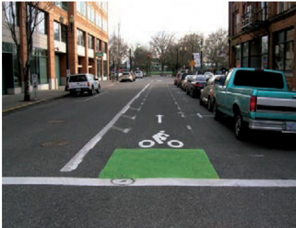
Figure 900-8: A striping buffer can be on the right or left of the bike lane.
