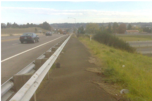
Figure 900-15: Guardrail in street buffer
