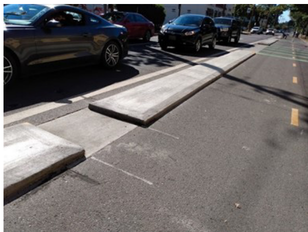
Figure 900-10: Island Buffer Cross Section with Drainage Gap
