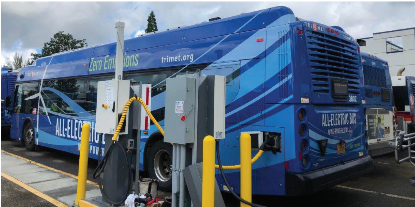
TriMet electric bus charging at a station, as part of a project with Portland General Electric.
