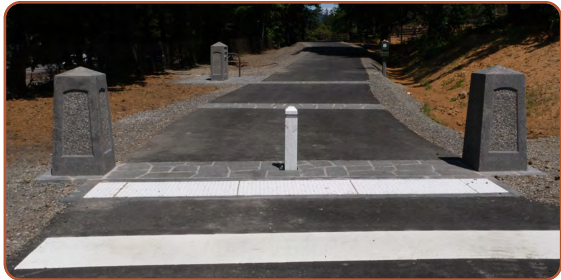
EXHIBIT 6: Recommended transition design. Existing transition at Viento Trailhead.
