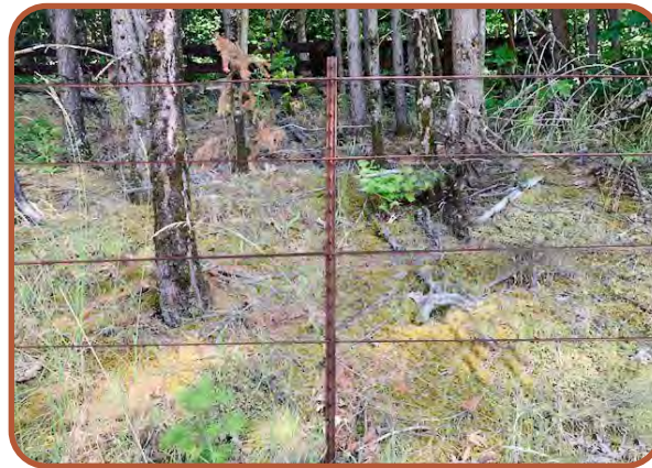
EXHIBIT 14: 4-wire fencing near Viento.
