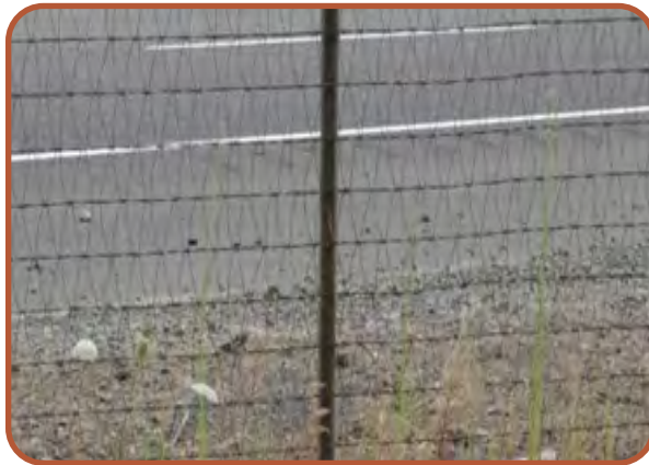
EXHIBIT 13: Existing V-Mesh fencing between Wyeth Trailhead and the Summit Creek Viaduct.
