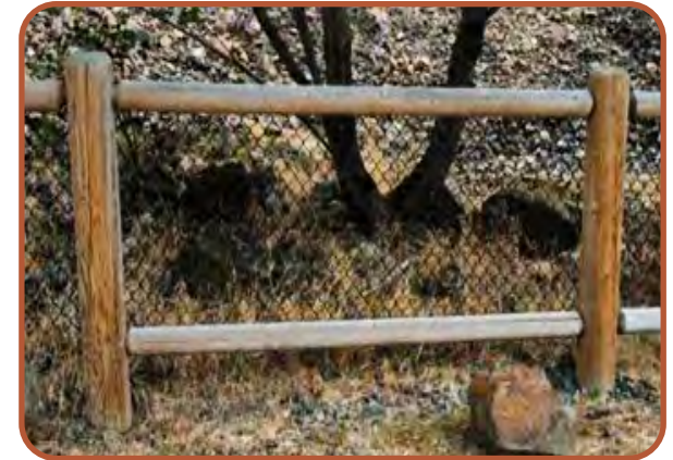
EXHIBIT 11: Existing access control fence in the Twin Tunnels section.
