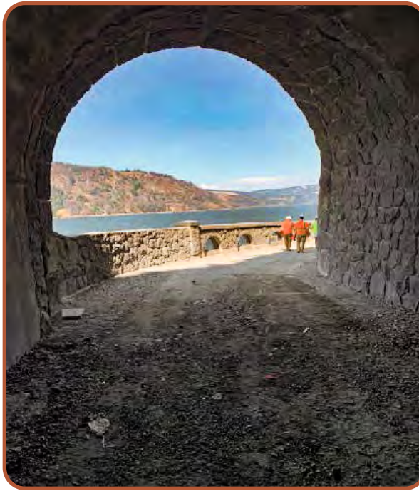
EXHIBIT 3: East Portal, Mitchell Point Tunnel.
