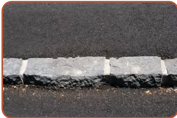
EXHIBIT 32: Recommended stone curb design. Existing stone curb at Viento Trailhead.
