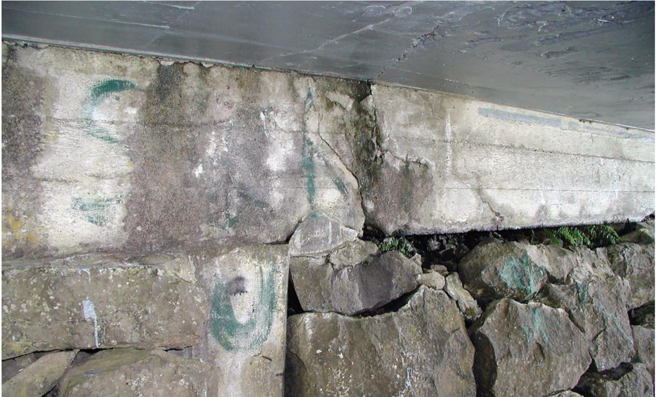
*Figure 77—Deterioration of the Crown Point Viaduct*
