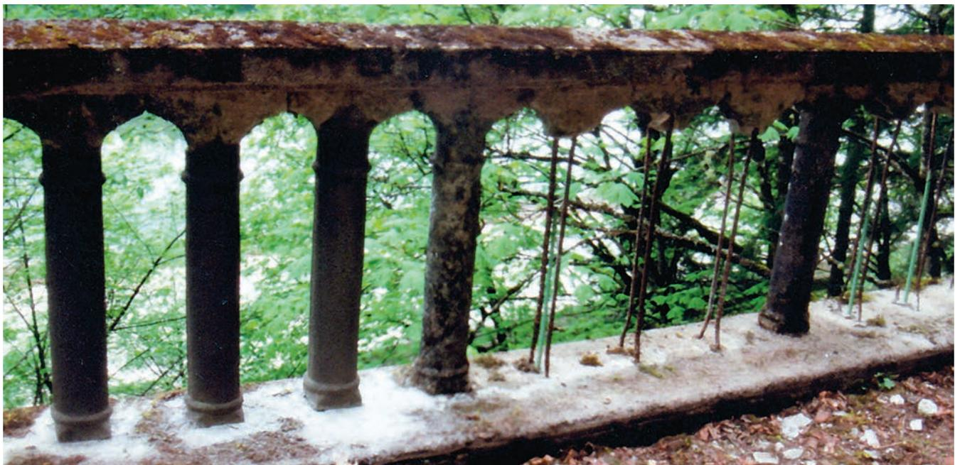
*Figure 79—Toothrock Viaduct Railing deteriorated Condition*
