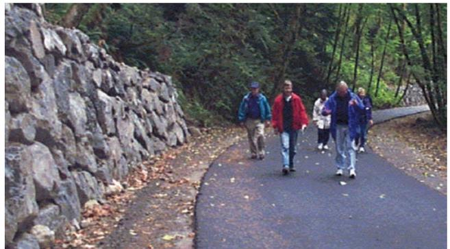
*Figure 106—Rockery retaining wall*
