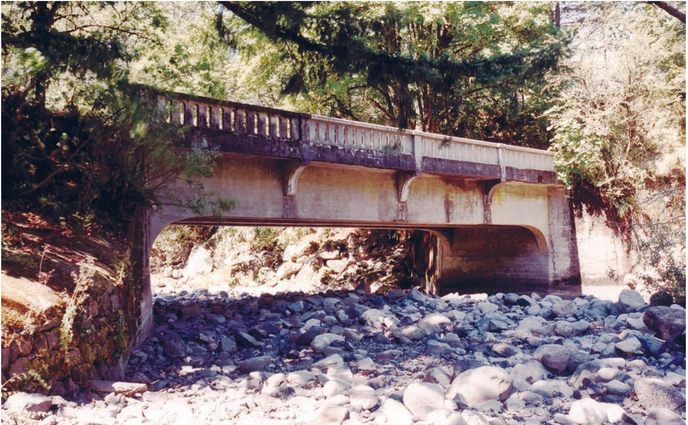
*Figure 102—Tanner Creek Bridge Railing Repaired*
