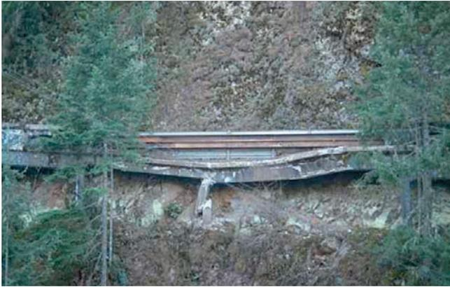
*Figure 80—Damaged Eagle Creek Viaduct*
