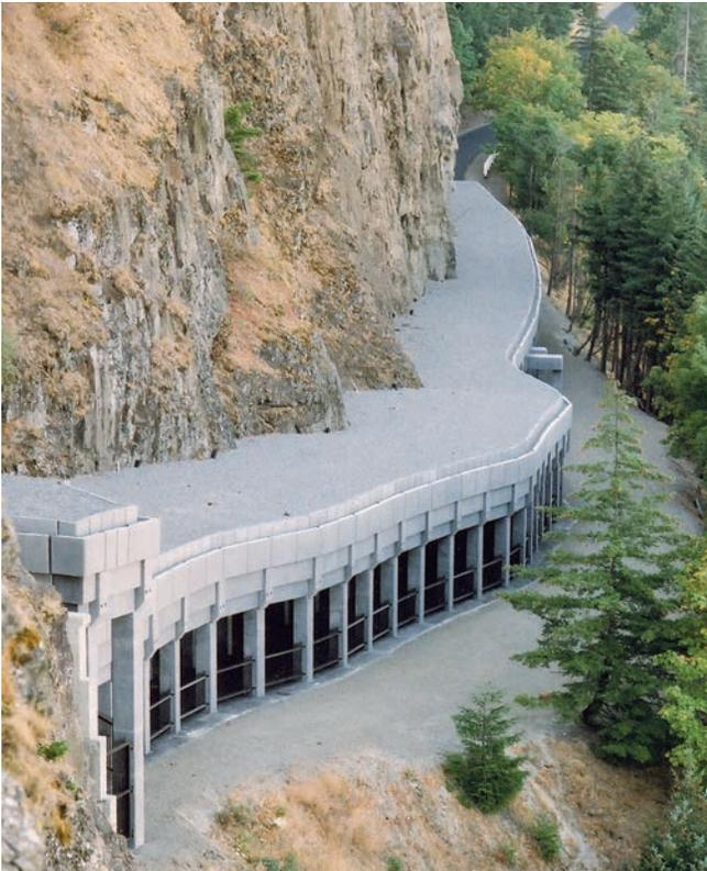
*Figure 89—Rockfall Catchment from Above*
