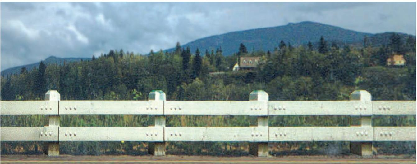
*Figure 61—Two-Rail, Steel-Backed, Wooden Guardrail*
