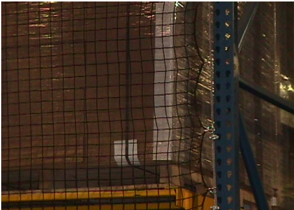
Figure 9. Rack netting at the Oregon Lottery warehouse.
