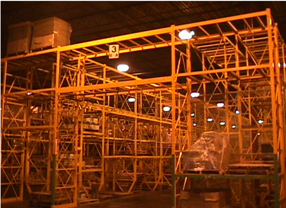
Figure 5. Racks on the main floor of the Department of Corrections warehouse connected by horizontal braces as well as bolted to the floor.
