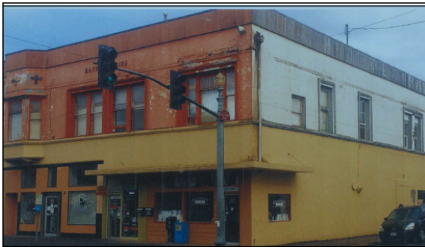
Bank Building Before Rehabilitation
