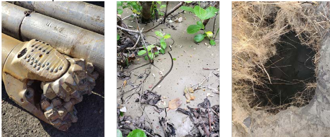
Figure 3: Drill bit, drilling fluid release, and sinkhole from previous projects.
