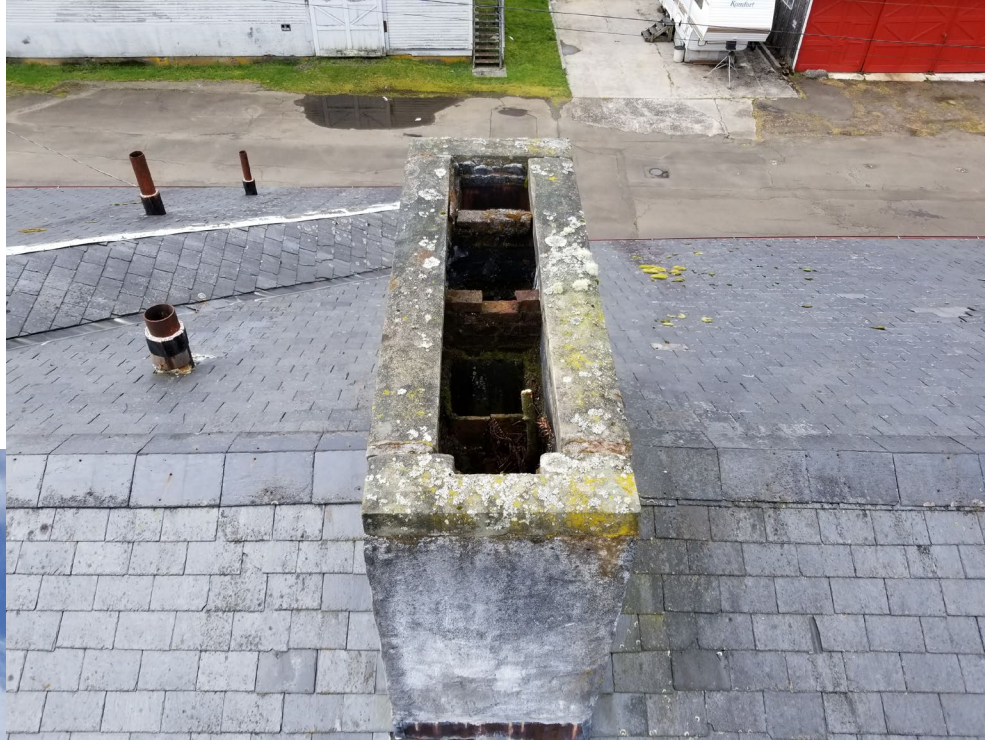
Chimney interior badly damaged.
