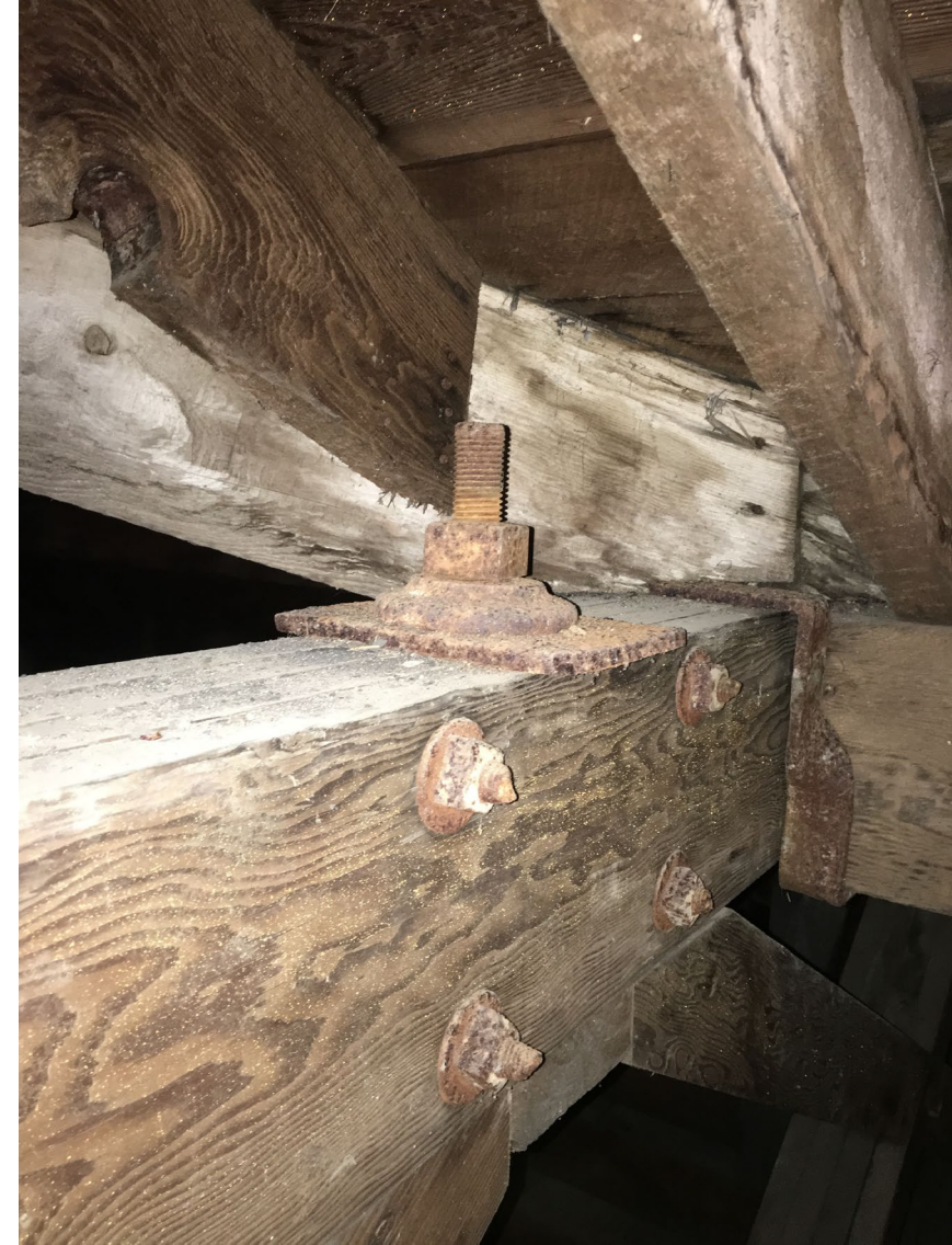
Water intrusion and white-rot fungi decay. Roof structure needs repaired to prevent collapse.
